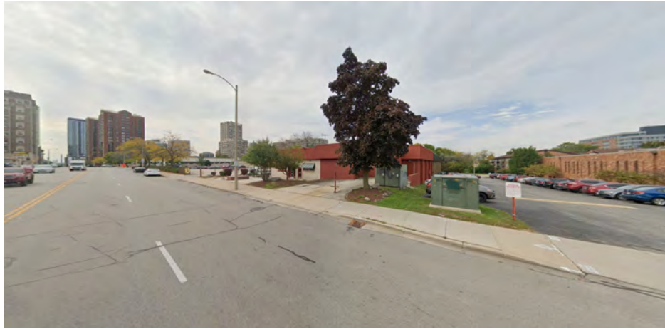
N/E Corner of Site - N Van Buren St, showing existing building
