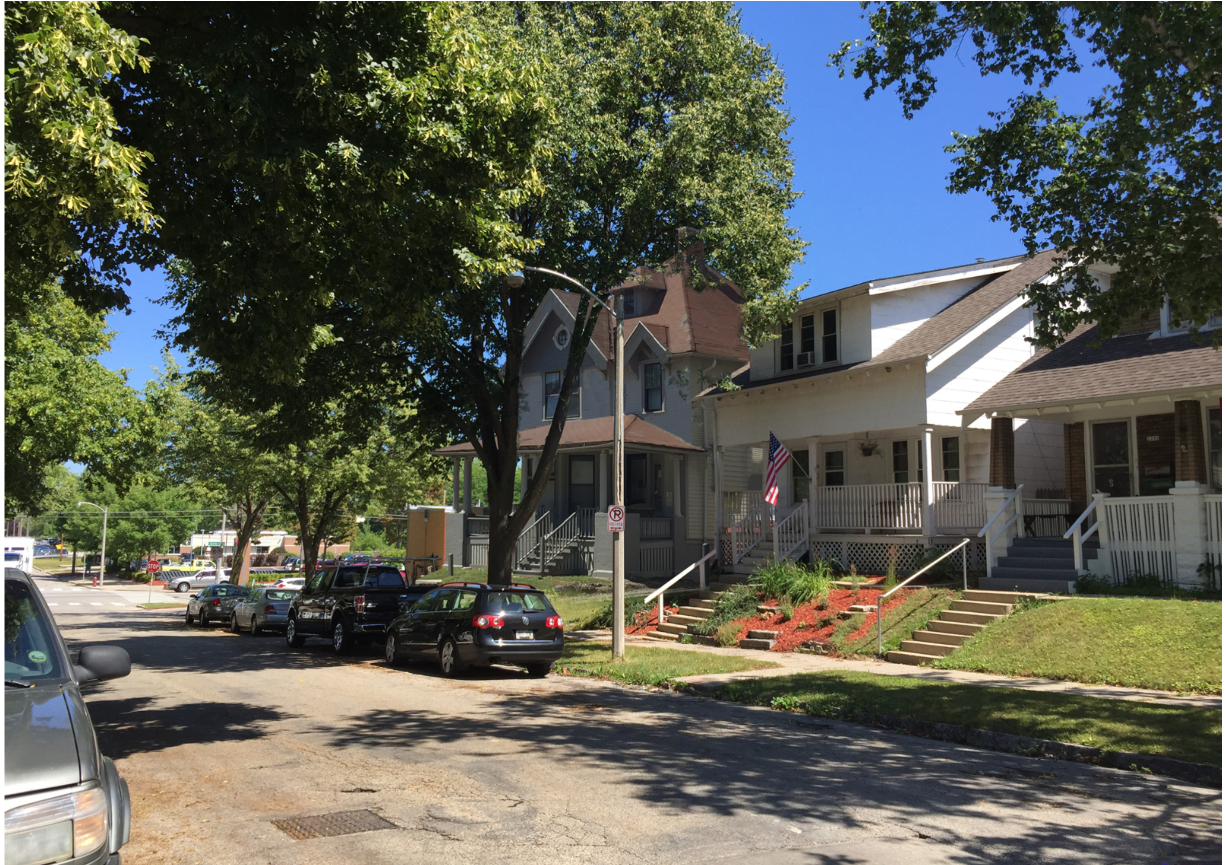
2208 NORTH NEWHALL : PROPOSED NEW LOCATION FOR CRAIN / CLAFLIN / ELDRED HOUSE (LOOKING NORTH ON NEWHALL)
