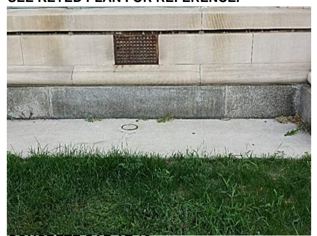
CONCRETE CAP AT 10
