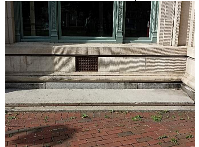
CONCRETE CAP AT 13
