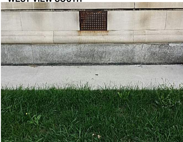
CONCRETE CAP, WEST EL
