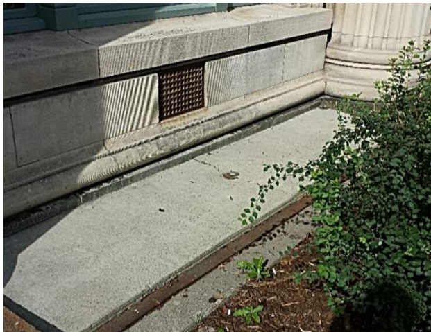
CONCRETE CAP AT 14
