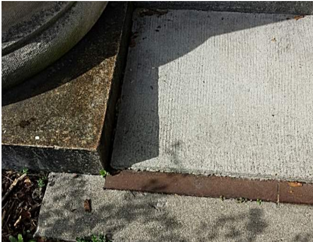
CONCRETE CAP AT 11
