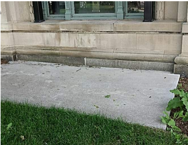
CONCRETE CAP AT NORTH END
