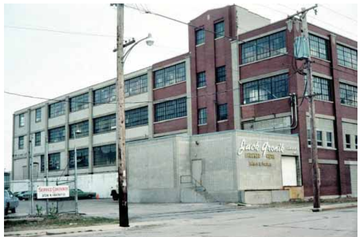
Figure 1.9 Older industrial building in Riverworks
