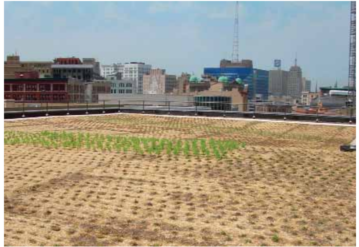
Figure 3.21 Department of City Development - Green Roof
