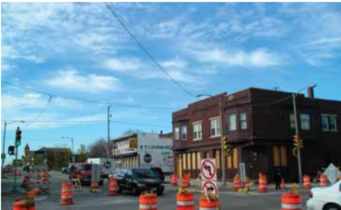
Figure 7.25: Center Street and Holton Street - Existing Conditions
