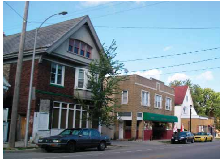
Figure 7.16: Center Street - Existing Streetscape Conditions
