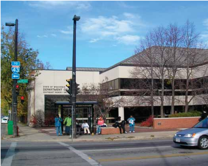
Figure 5.32: DNR Building and site to be Redeveloped
