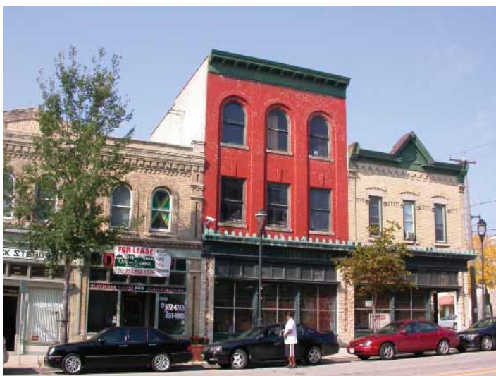
Figure 5.6: Historic King Drive
