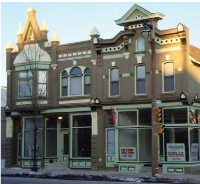
Figure 5.34: Historic Building after facade renovation.
