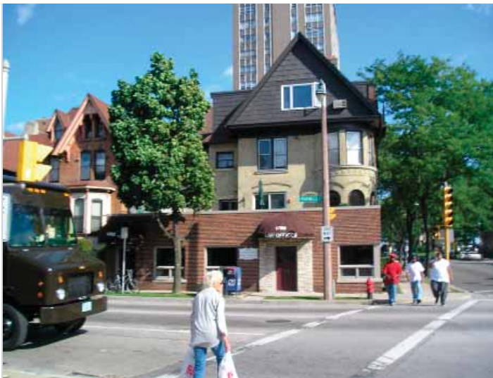
Figure 10.16: Farwell Avenue Looking East
