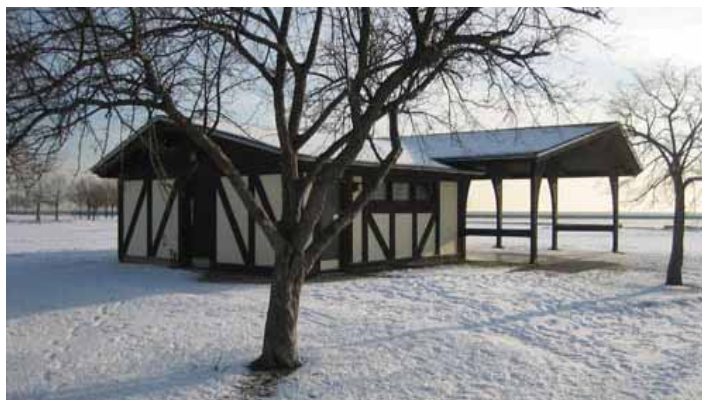
Figure 11.30: Existing Restrooms and Picnic Pavilion
