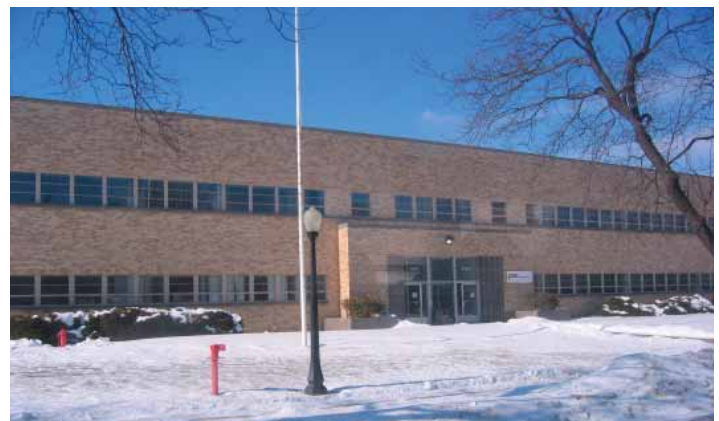
Figure 6.4: Existing Industrial Buildings
