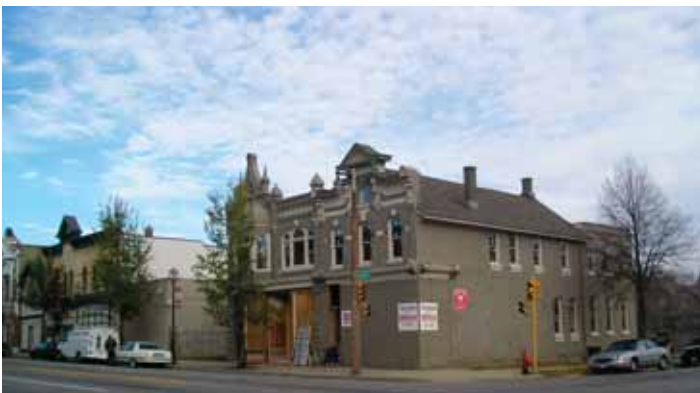
Figure 7.26: Center Street and Holton Street - Existing Conditions
