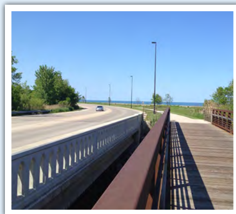
Surface Arterial (STH 32) in Kenosha Credit: SEWRPC
