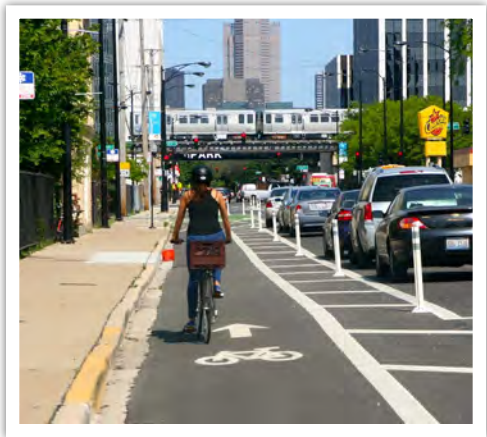
Protected Bike Lane with Bollards in Chicago Credit: People for Bikes
