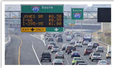
Tolls with Pricing Based on Congestion Level Credit: Minnesota Department of Transportation
