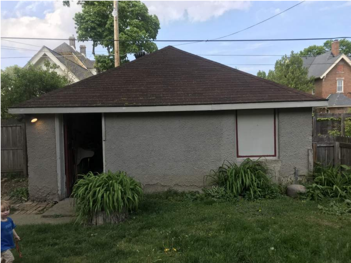
Photo 4 - South Elevation of the Existing Garage
