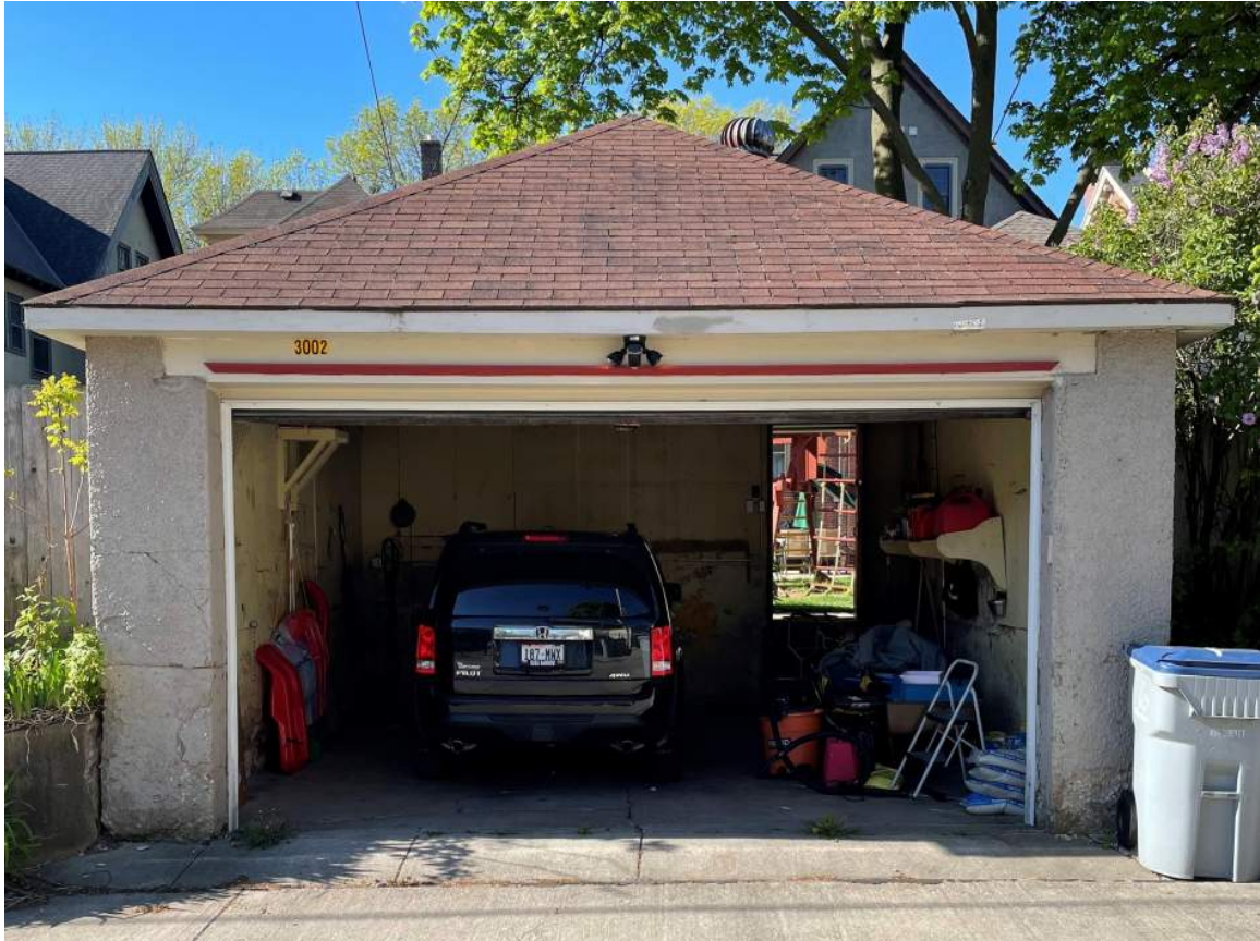
Photo 5 - North Elevation of the Existing Garage
