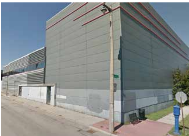
The former Almacenes El Rey at 7th and National has been marketed for sale and is ripe for redevelopment. (Source: Google Streetview)
