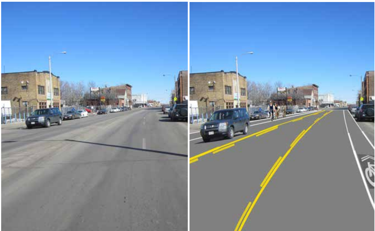
Example of the existing National Avenue configuration and a potential three-lane configuration with bike lanes. (Source: DCD / Planning)
