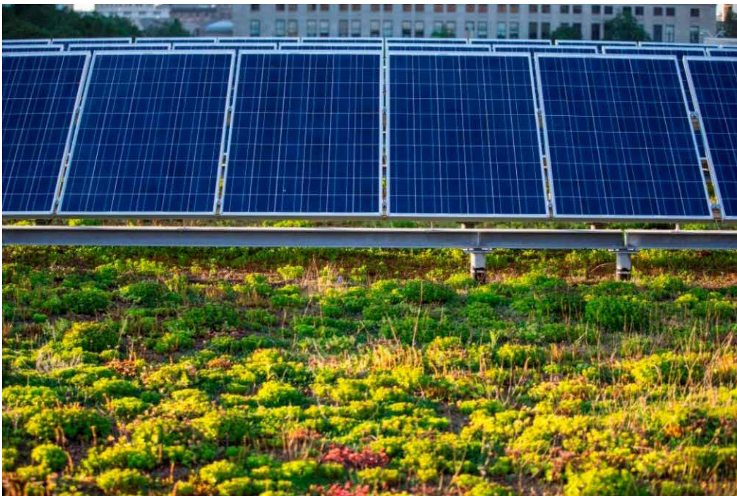
Milwaukee Public Library's Green Roof.
