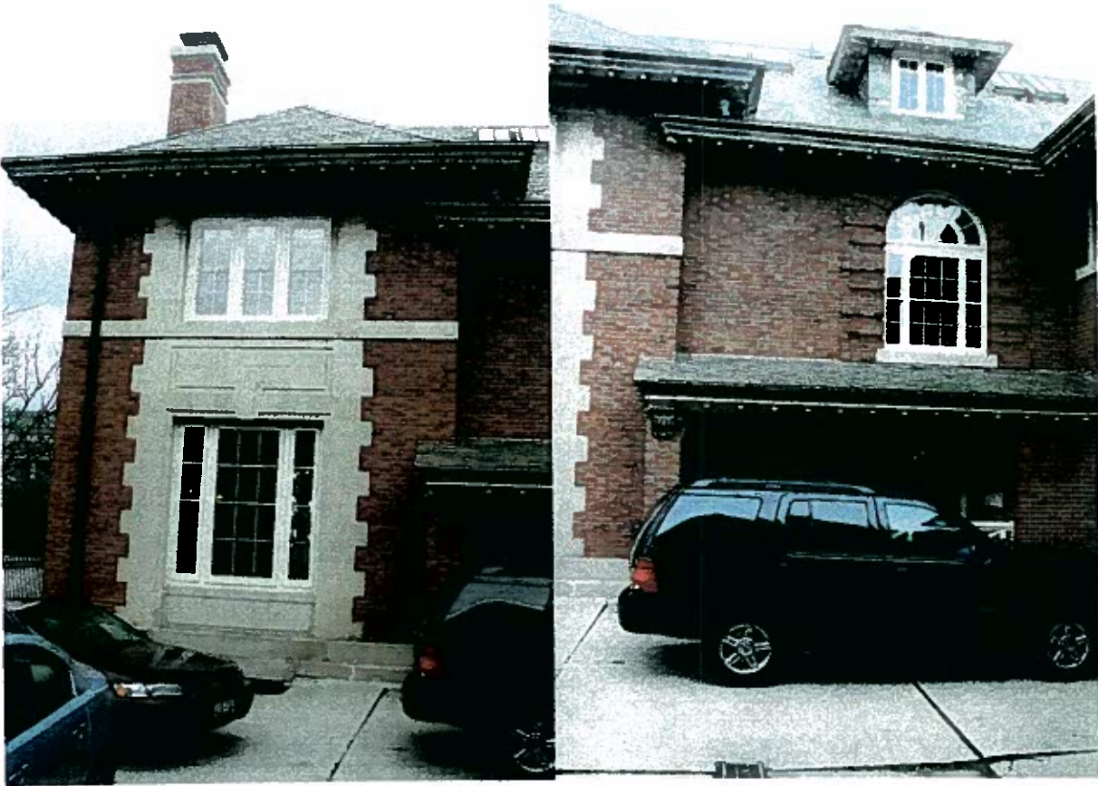
Main House Elevation (west) – From Driveway
