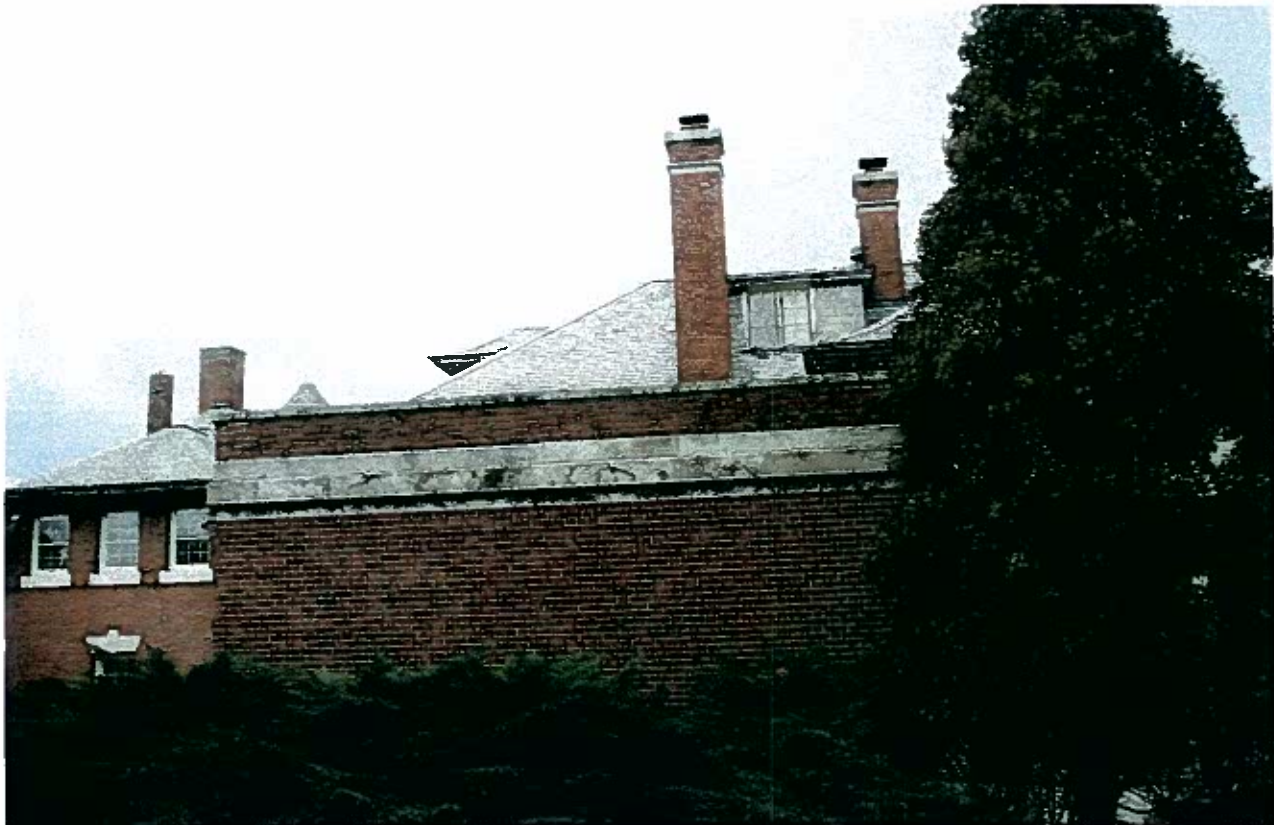
Main House Elevation(south) – from backyard
