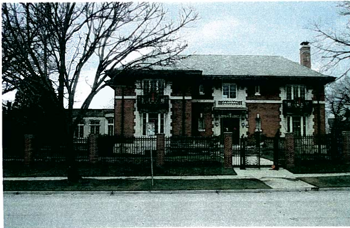
Main House Elevation(east) - from North Terrace Avenue
