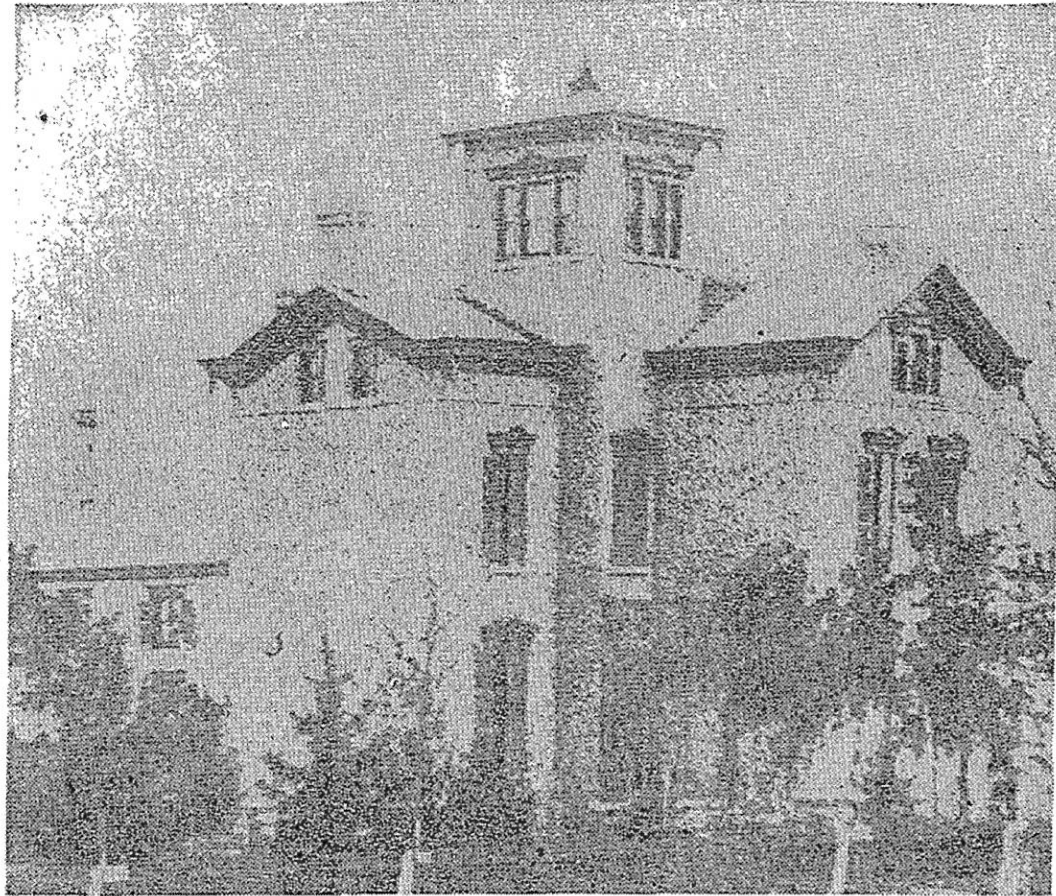
This 1870-'90 era photo shows the Aring home in its original form
