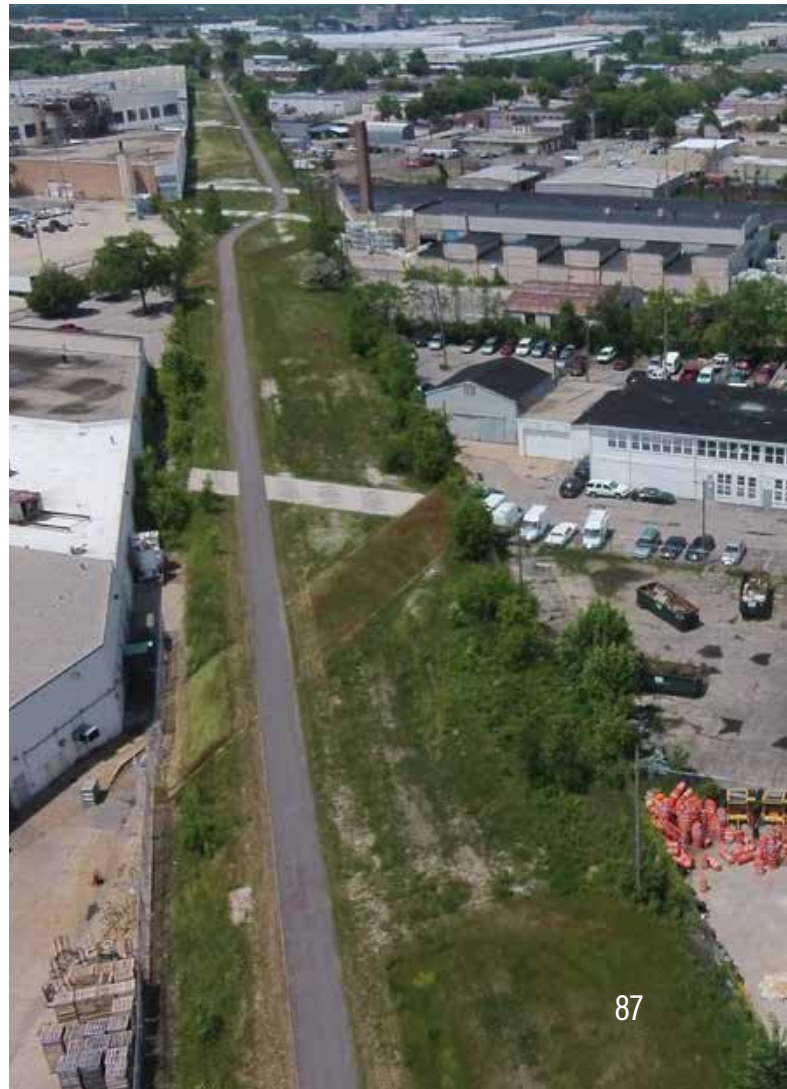
► Existing conditions of the B-Line, courtesy of Hood Design Studios
