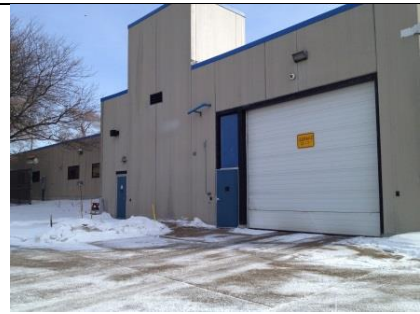
Rear Loading Dock Entrance
