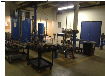
Large Meter Testing Facility
