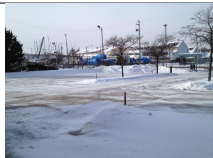
Rear Parking Lot
