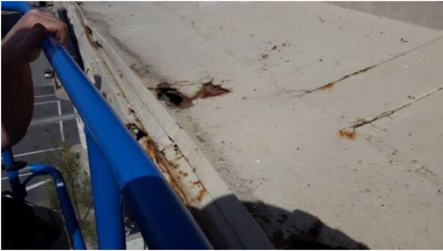
Photos 5, 6 – Corroded formed, painted metal cornice trim. South elevation, western-end.
