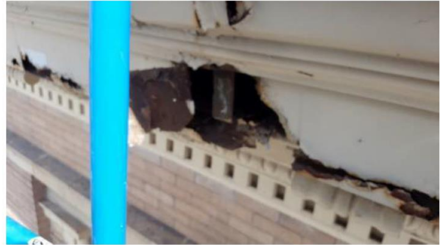
Photos 5, 6 – Corroded formed, painted metal cornice trim. South elevation, western-end.
