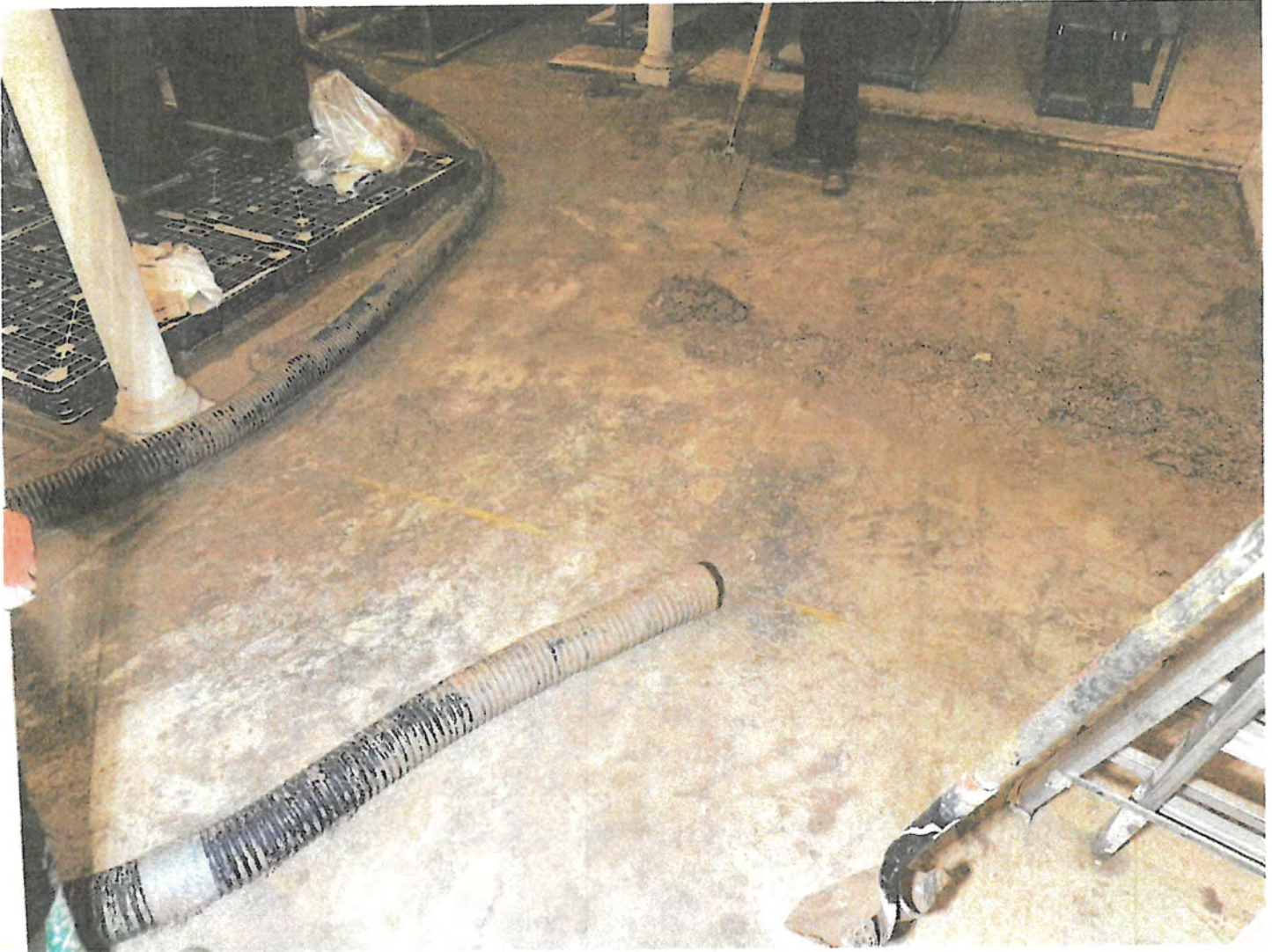
62 62-Environmental company removing the sludge.
