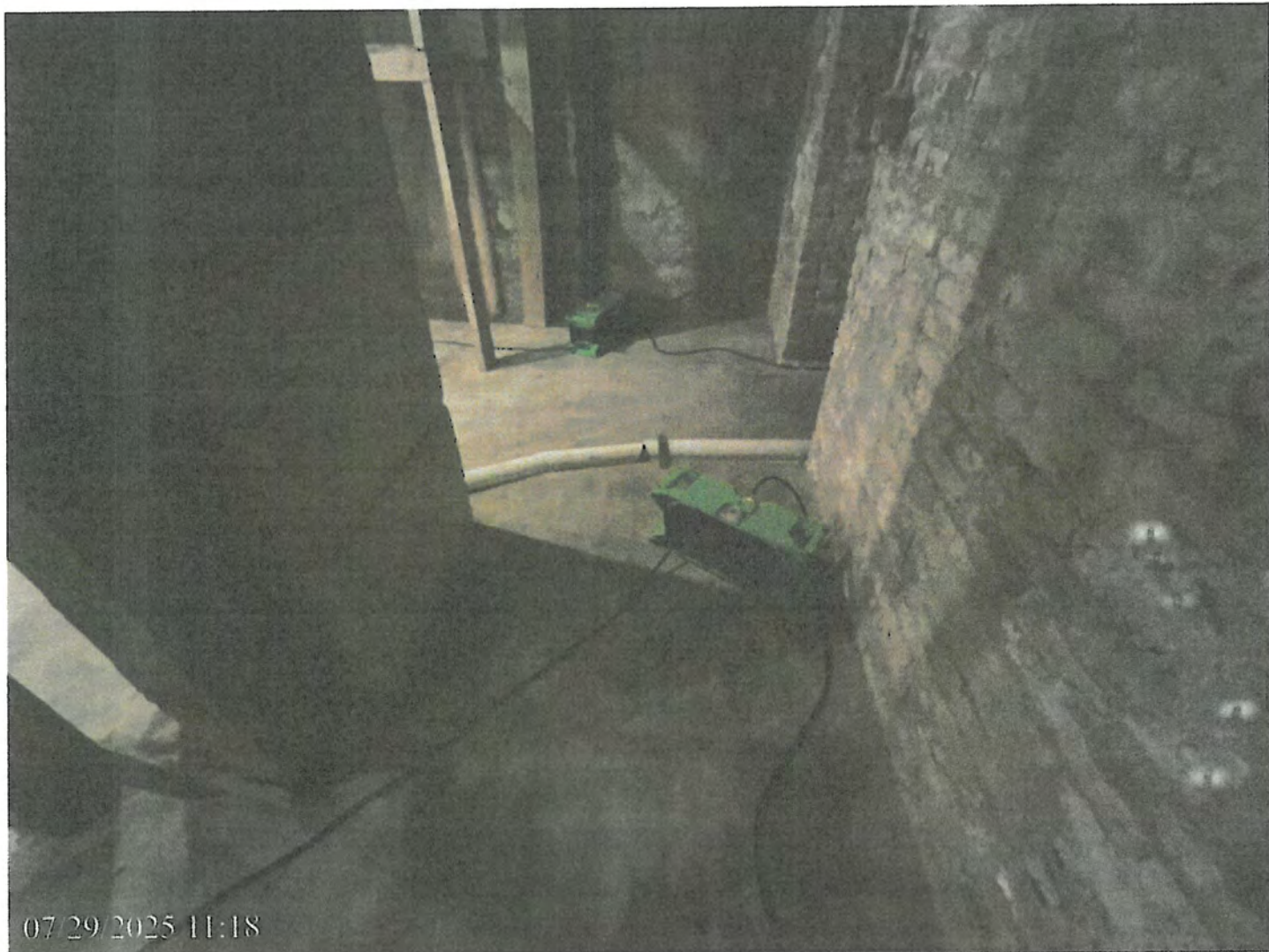
20 20-2 air movers in Basement on 7_ Date Taken: 7/29/2025 29, placed on 7
