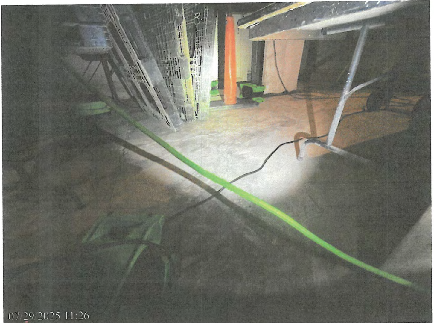
48 48-5 air movers Under Stairs on 7_ Date Taken: 7/29/2025 29, placed on
