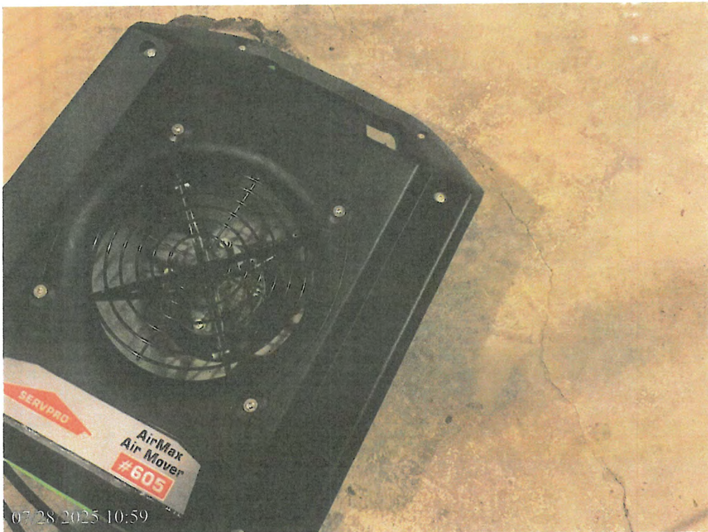
4 4-1 air mover in Basement on 7_ Date Taken: 7/28/2025 28, placed on 7_
