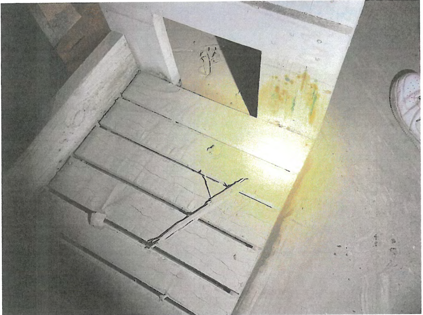
98 98-Visible potential microbial growth. 2
