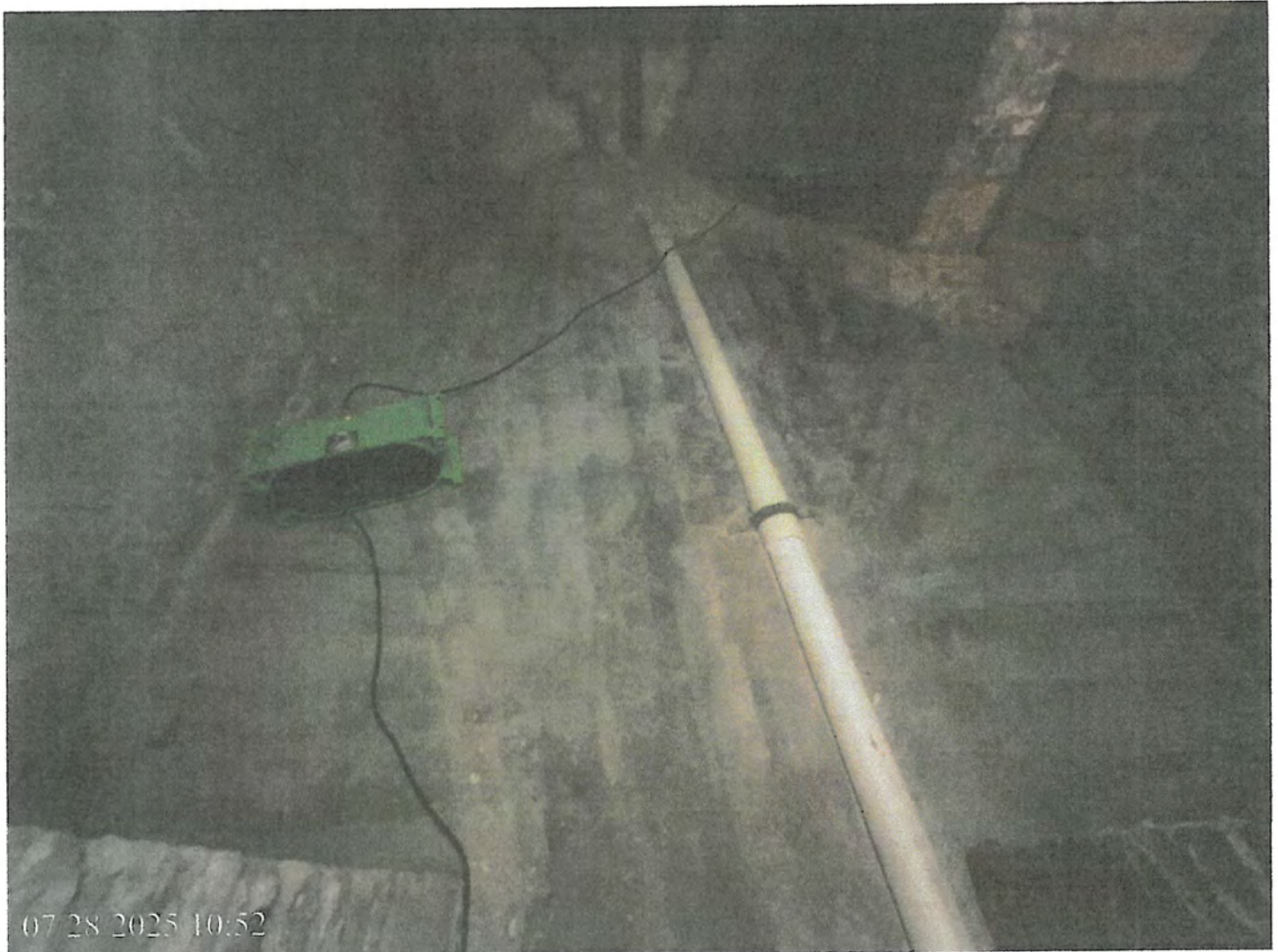
22 22-2 air movers in Left Catacombs Date Taken: 7/28/2025 on 7_28, place
