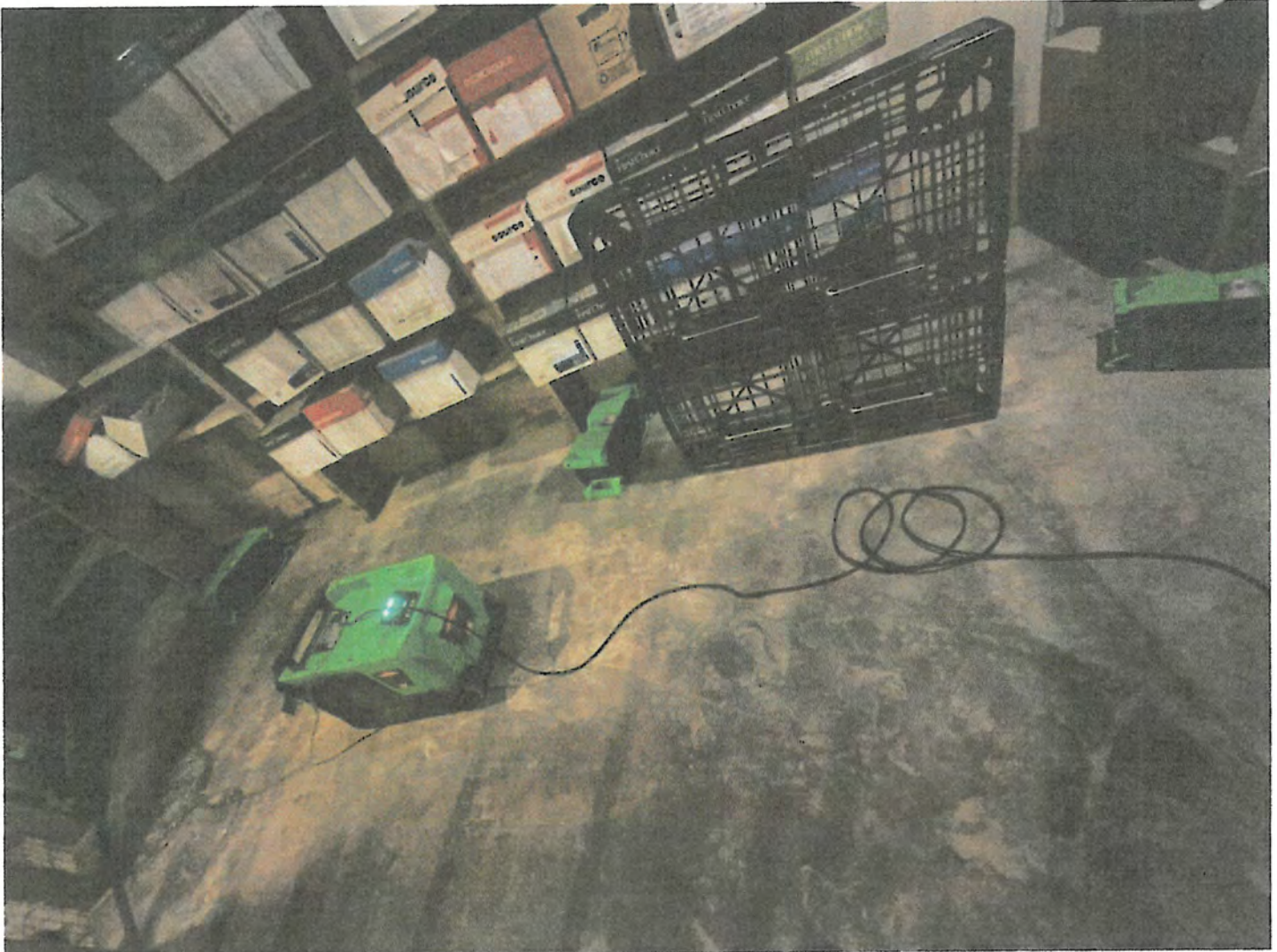
37 37-4 air movers & 1 dehu in Basement Storage.
