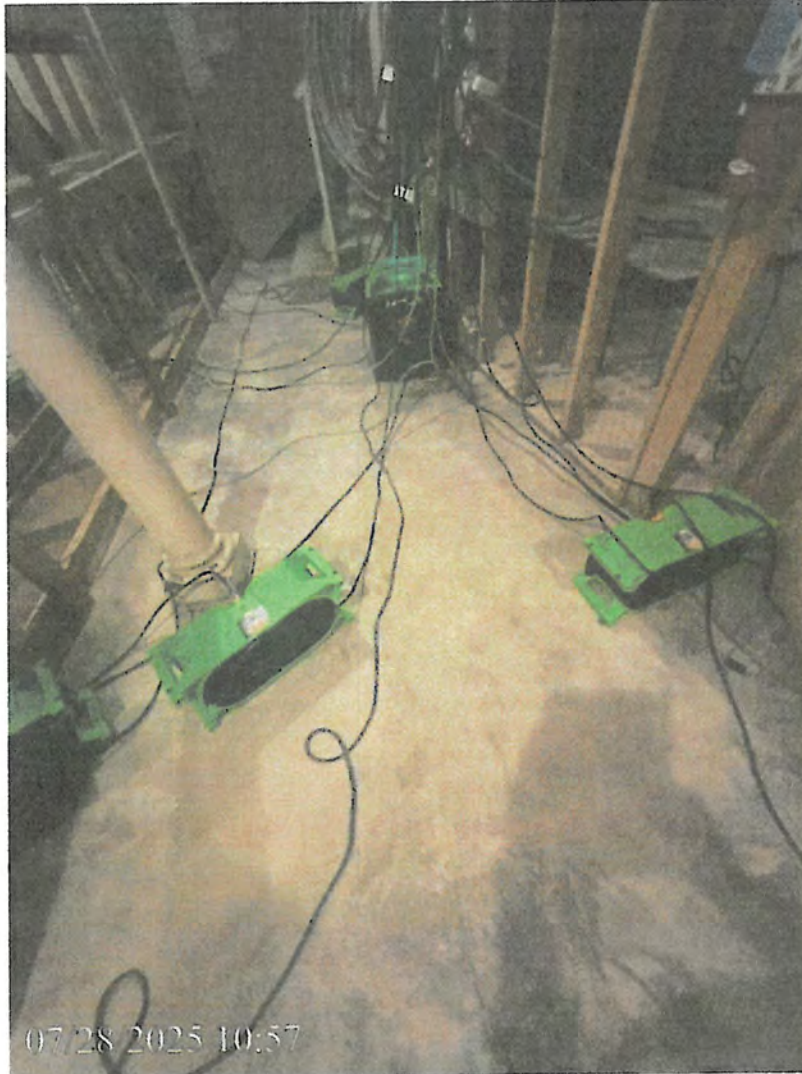
49 49-5 air movers, 1 dehu, & 1 temp panel in Basem Date Taken: 7/28/2025
