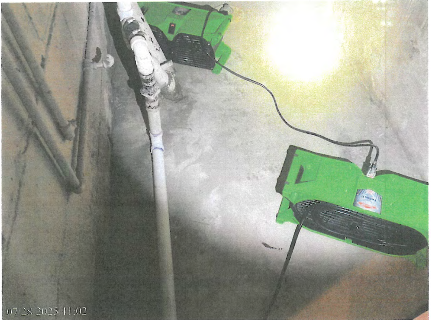
16 16-2 air movers in Basement Closet Date Taken: 7/28/2025 on 7_28, plac
