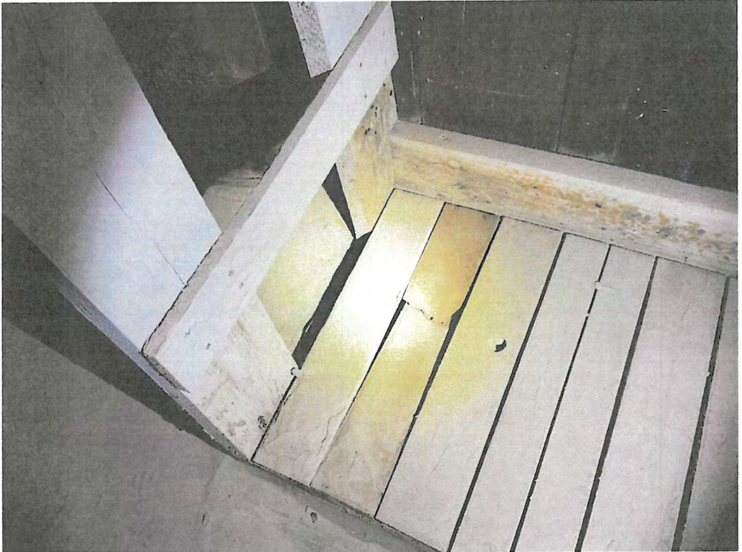
100 100-Visible potential microbial growth. 4
