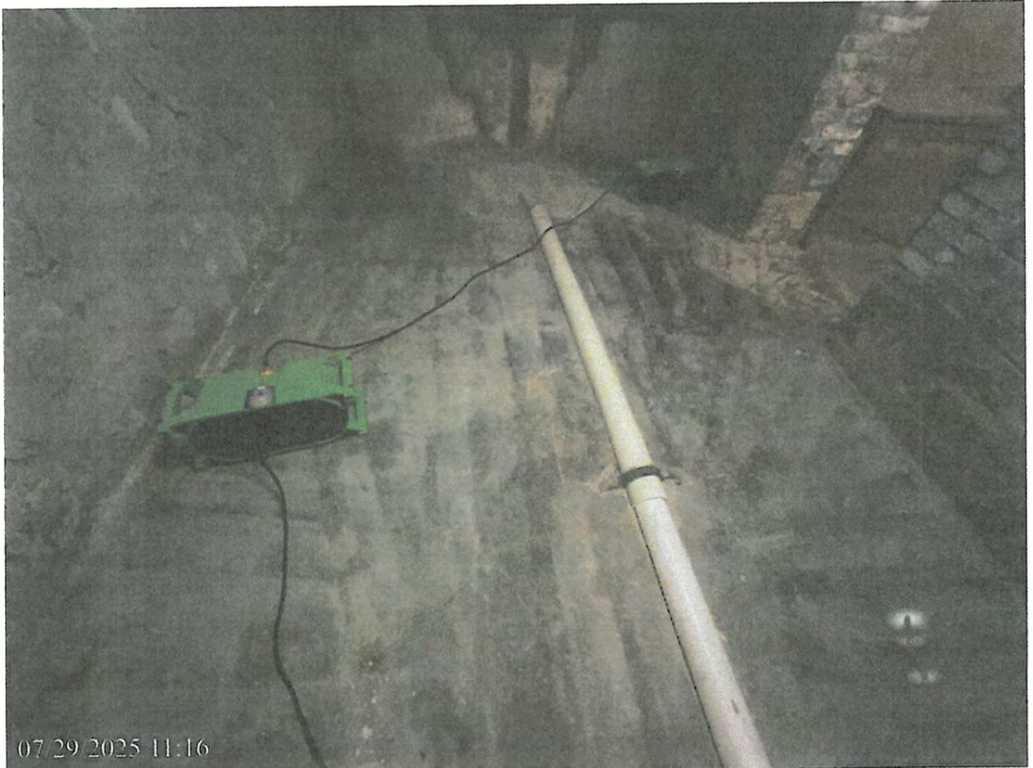
23 23-2 air movers in Left Catacombs Date Taken: 7/29/2025 on 7_29, place
