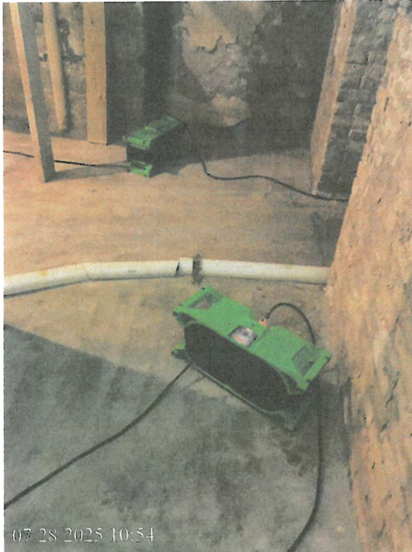
19 19-2 air movers in Basement on 7_ Date Taken: 7/28/2025 28, placed on 7
