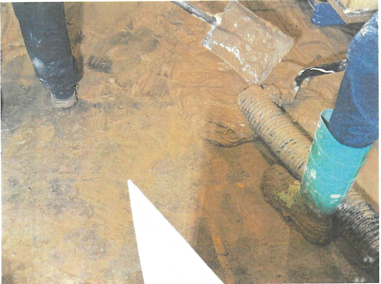
61 61-Environmental company removing the sludge. 2
