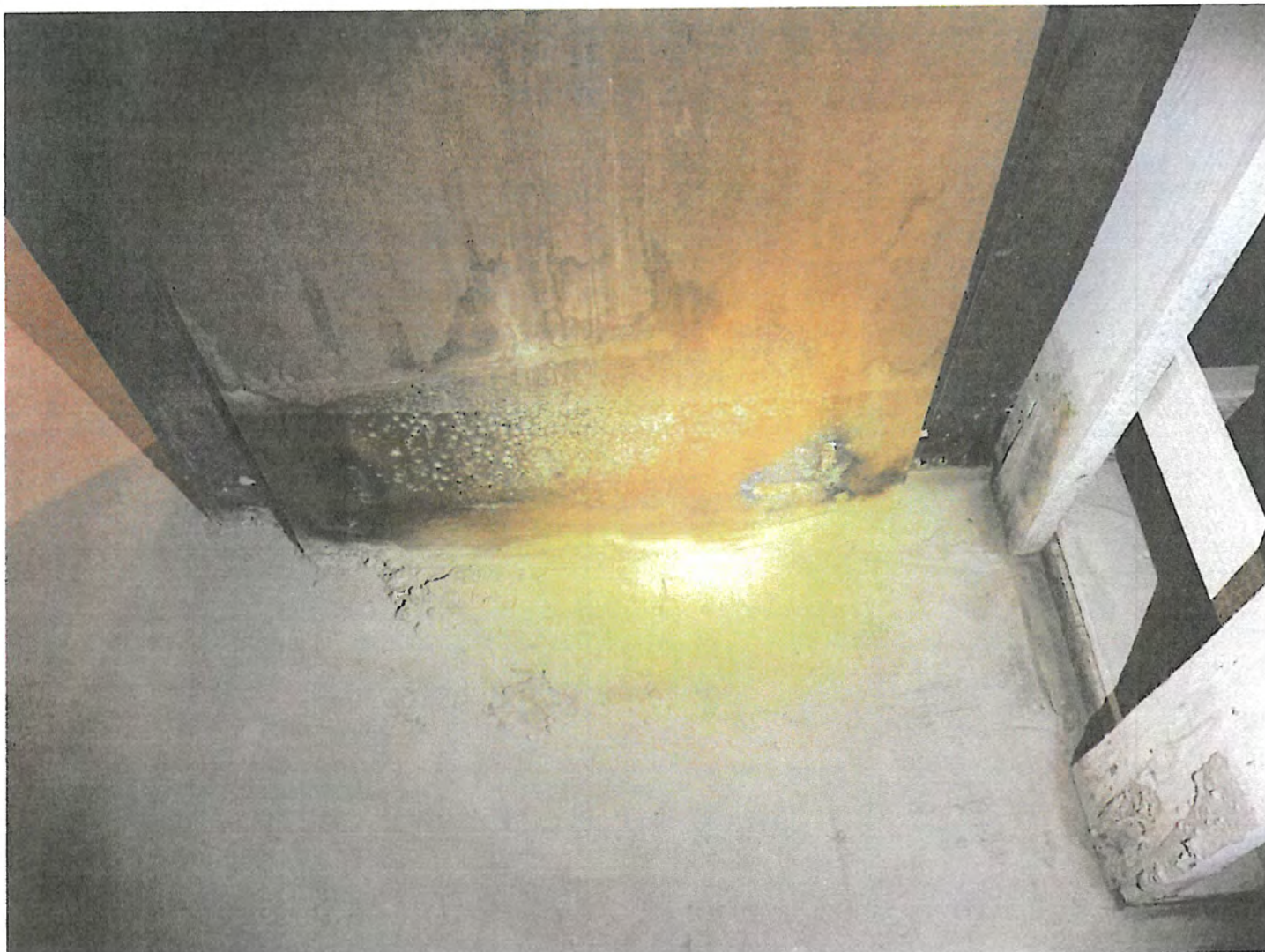
103 103-Visible potential microbial growth. Date Taken: 7/21/2025
