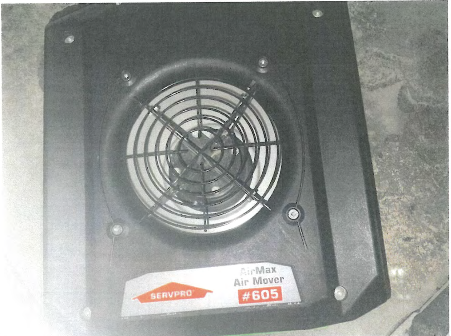
11 11-1 more air mover in Basement. Date Taken: 7/28/2025
