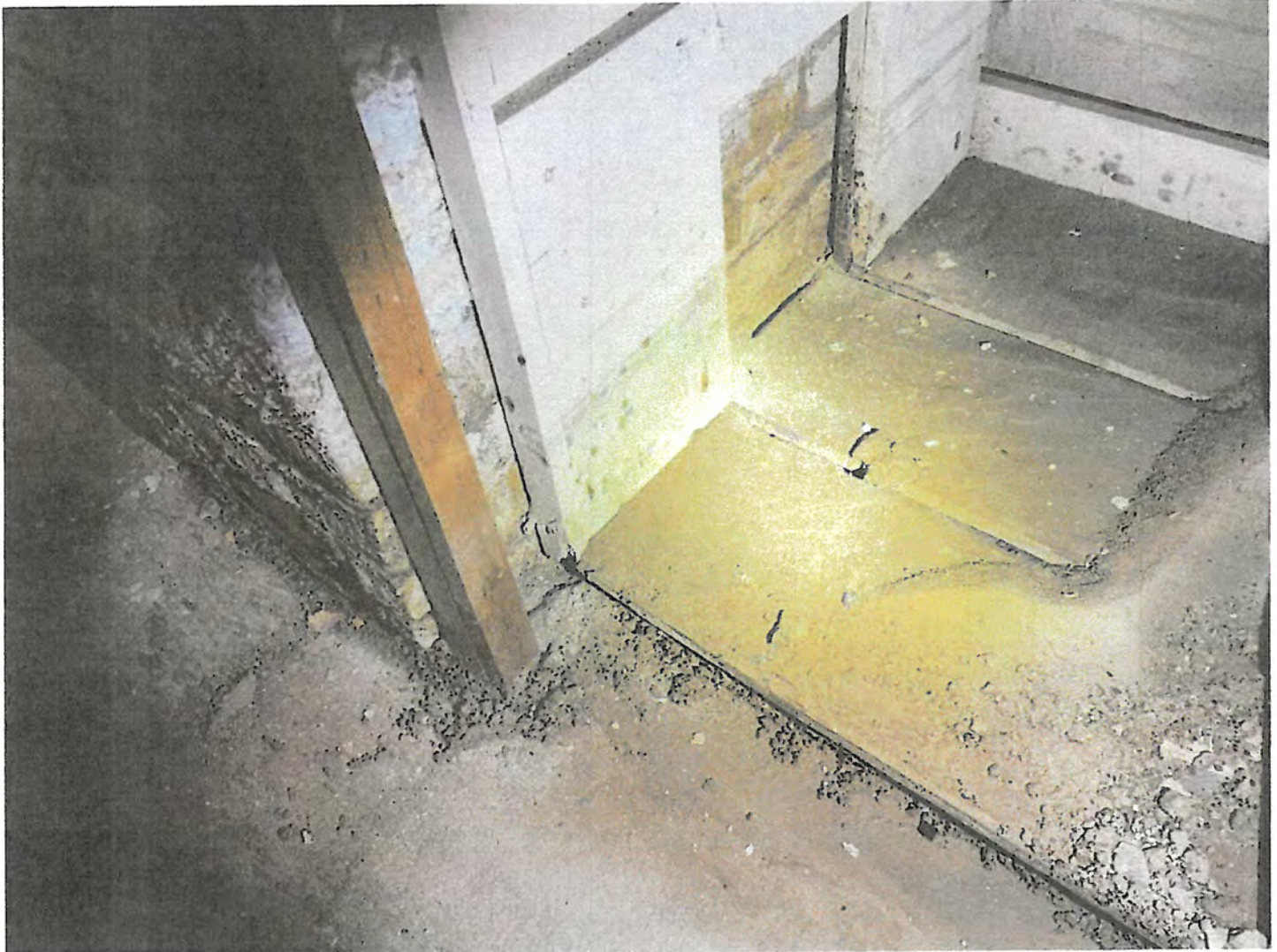
102 102-Visible potential microbial growth. 6 Date Taken: 7/21/2025
