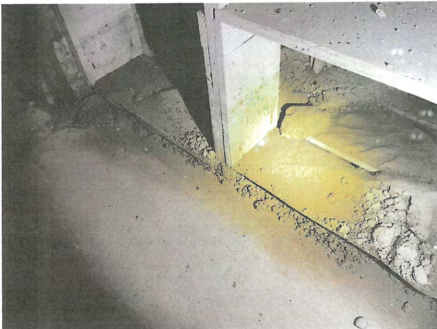
101 101-Visible potential microbial growth. 5 Date Taken: 7/21/2025
