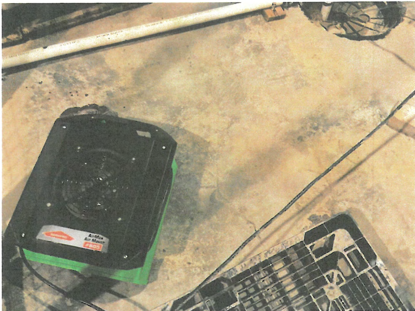
3 3-1 air mover in Basement Hallway. Date Taken: 7/25/2025
