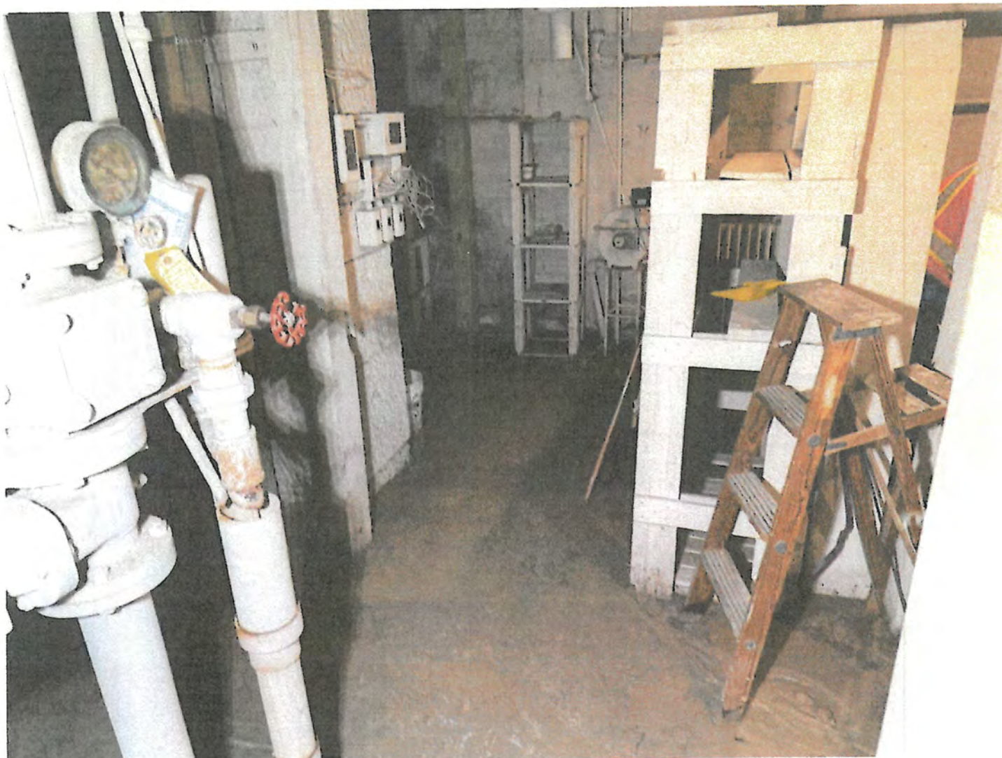
56 56-After environmental company removed the sludge Date Taken: 7/15/2025
