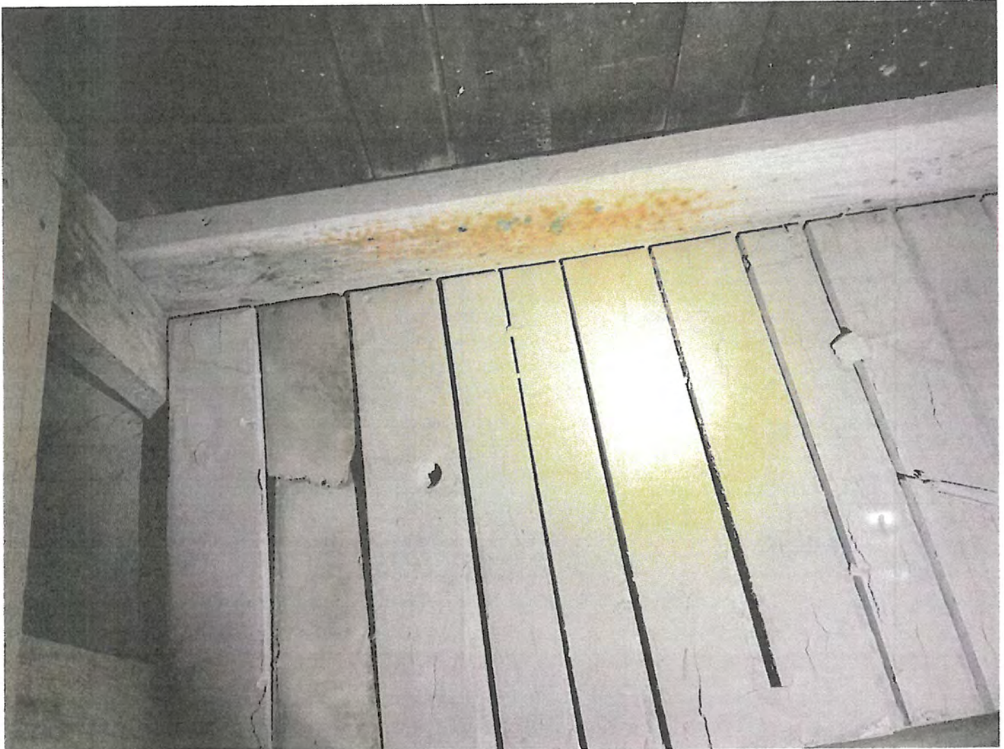
99 99-Visible potential microbial growth. 3
