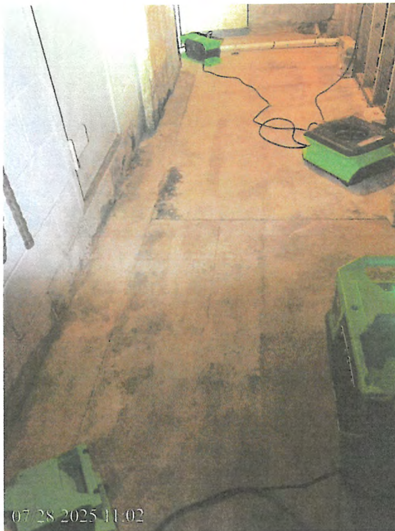
34 34-3 air movers Under Stairs on 7_ Date Taken: 7/28/2025 28, placed on
