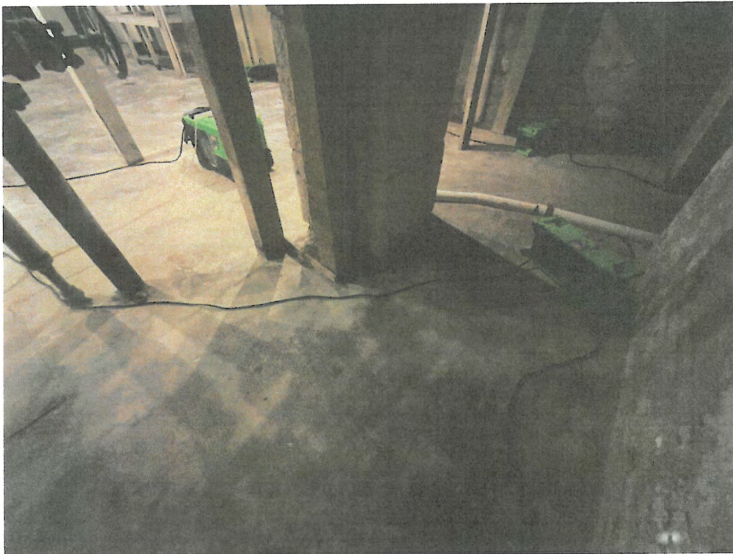
39 39-4 air movers & 1 dehu in Basement.
