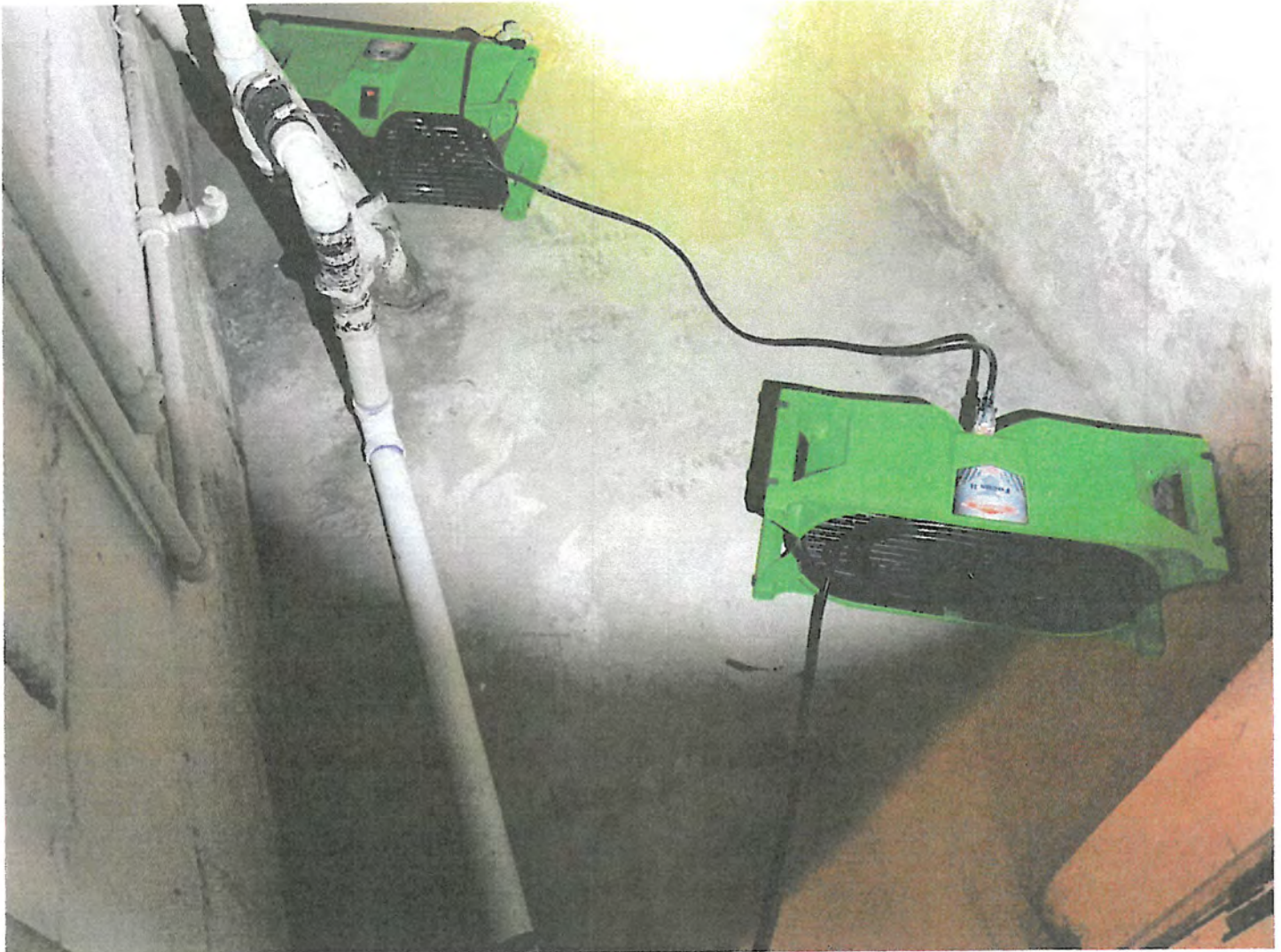
18 18-2 air movers in Basement Closet. Date Taken: 7/25/2025
