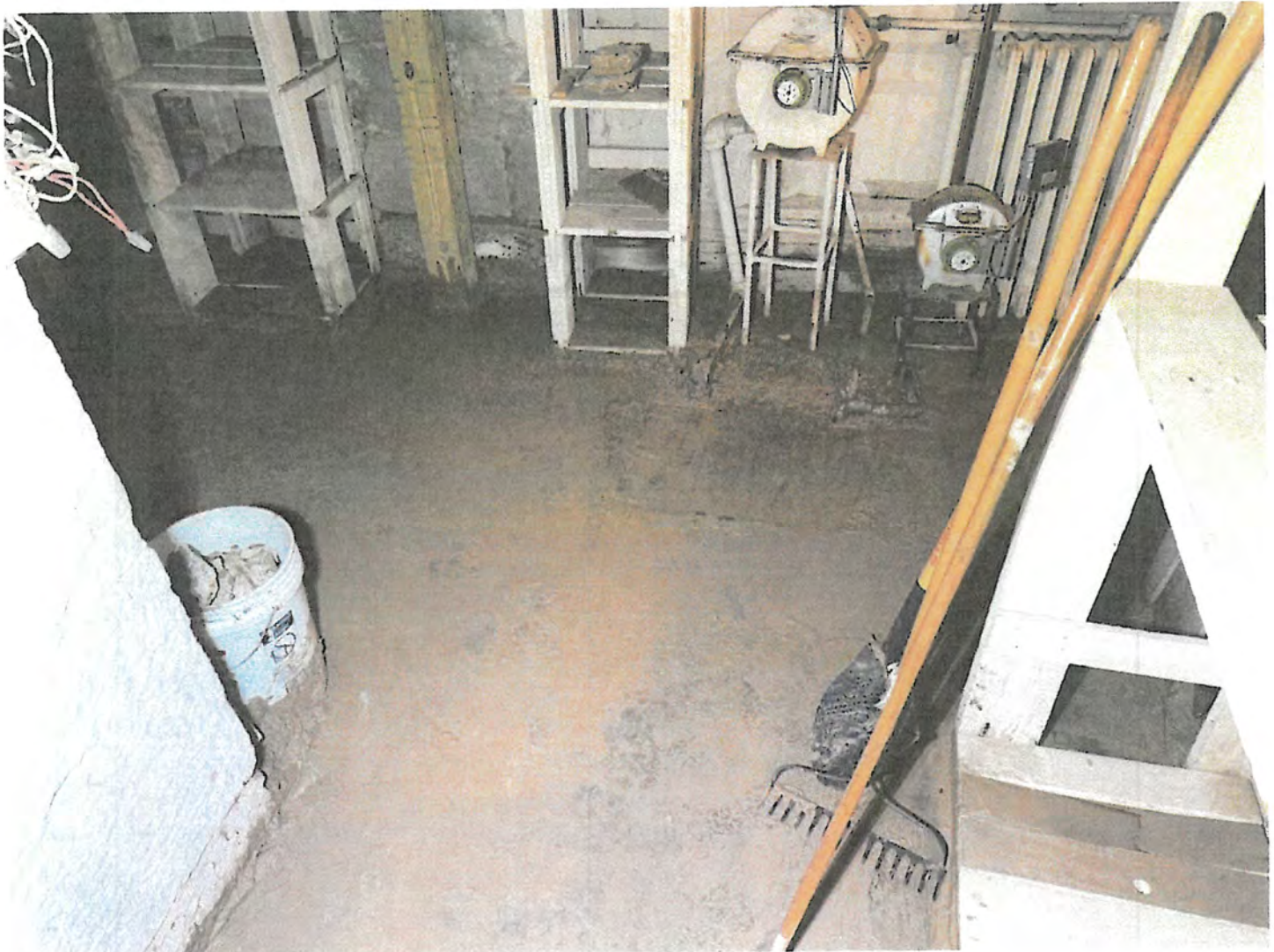
57 57-After environmental company removed the sludge Date Taken: 7/15/2025
