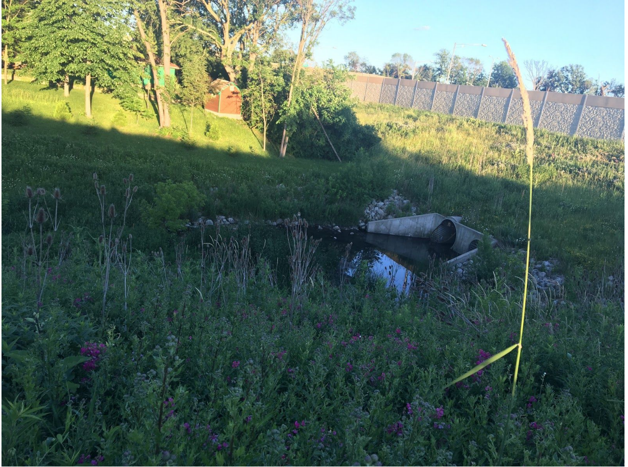
East View Facing Drainage Channel
