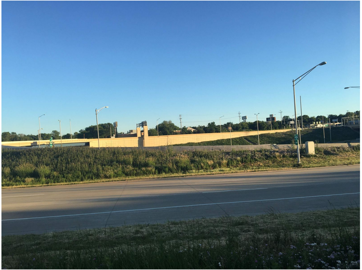
South View Facing The Highway Ramp
