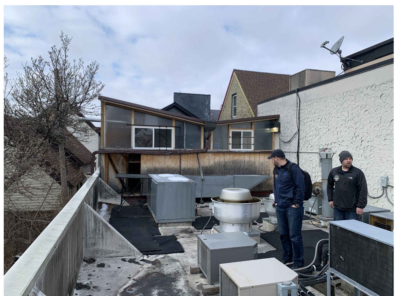
Photo East Lower Roof SCALE: NO SCALE
