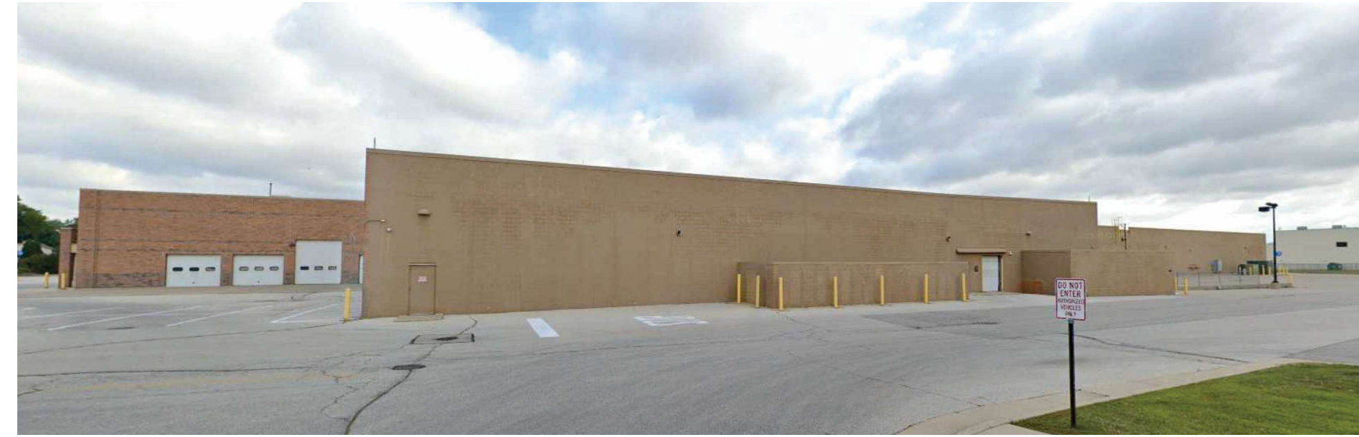
SOUTH SIDE OF EXISTING BUILDING
