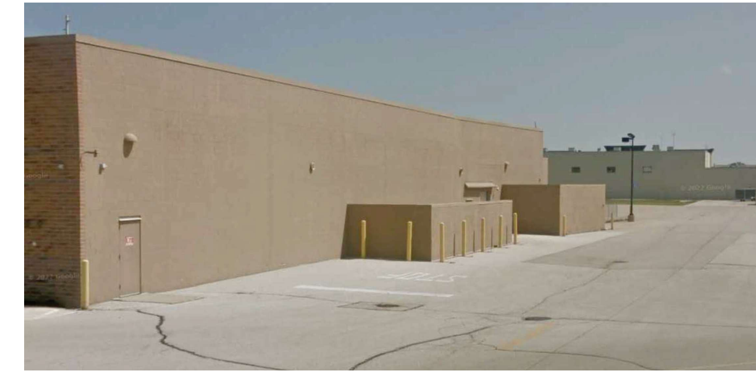
SOUTH SIDE OF EXISTING BUILDING
