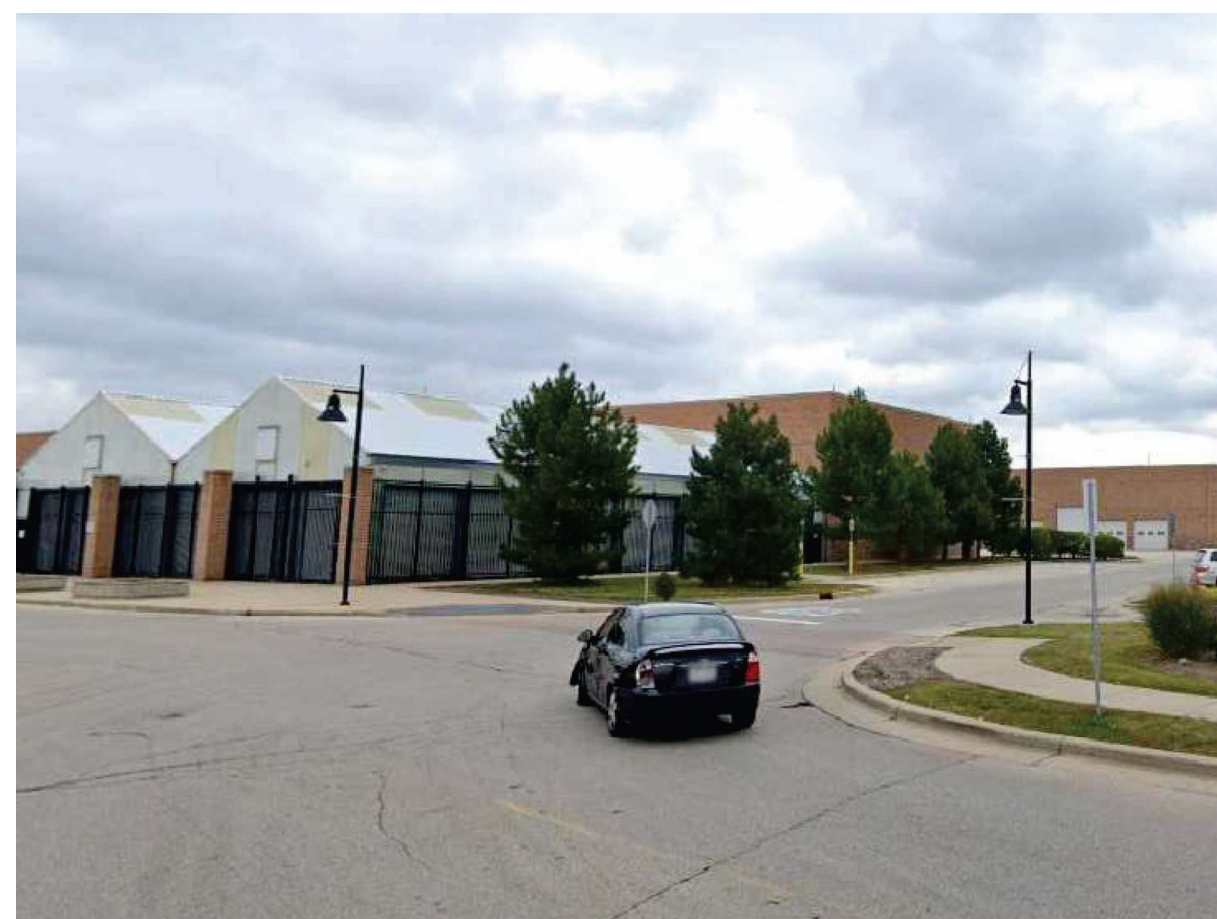
NORTHWEST SIDE OF BUILDING - EXISTING GREENHOUSES
