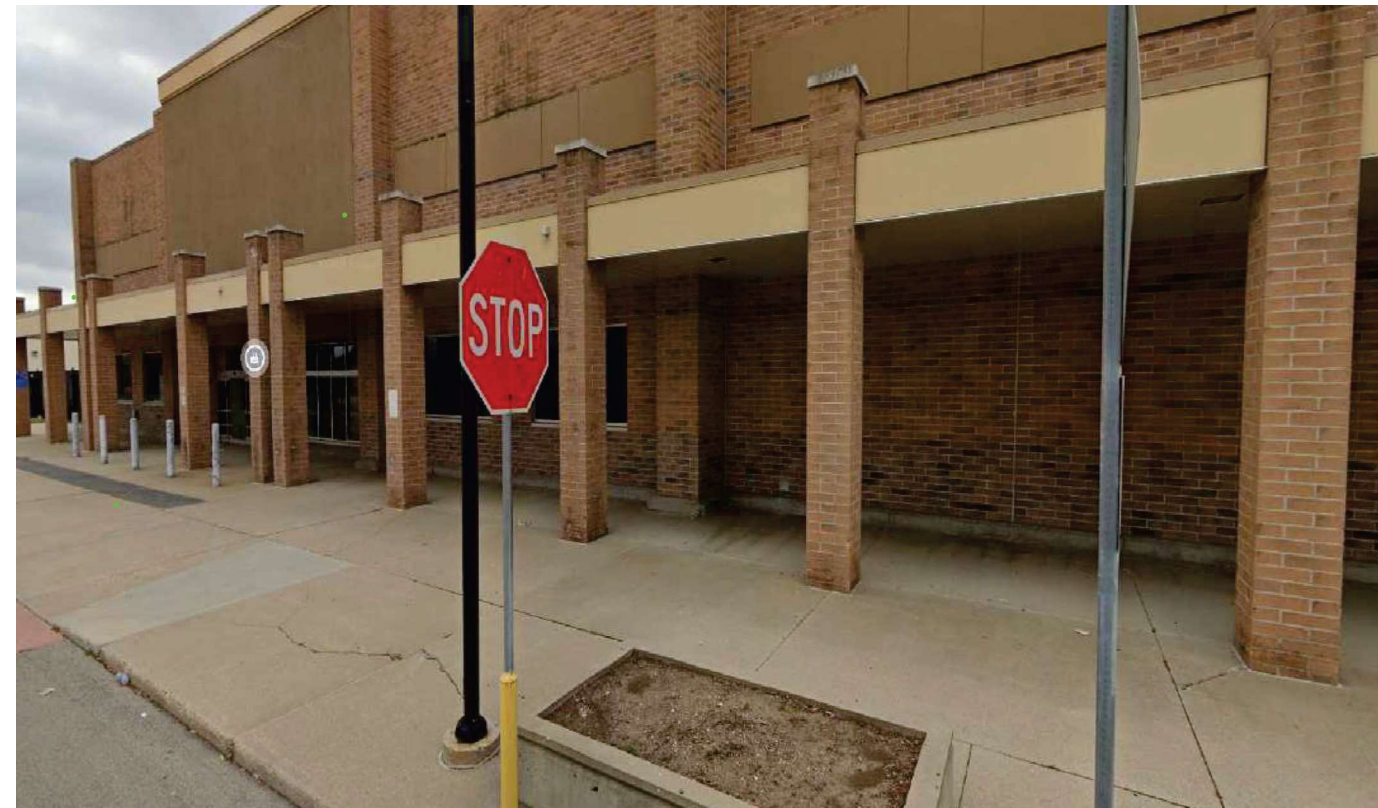
NORTH SIDE OF EXISTING BUILDING - FORMER WALMART ENTRANCE
