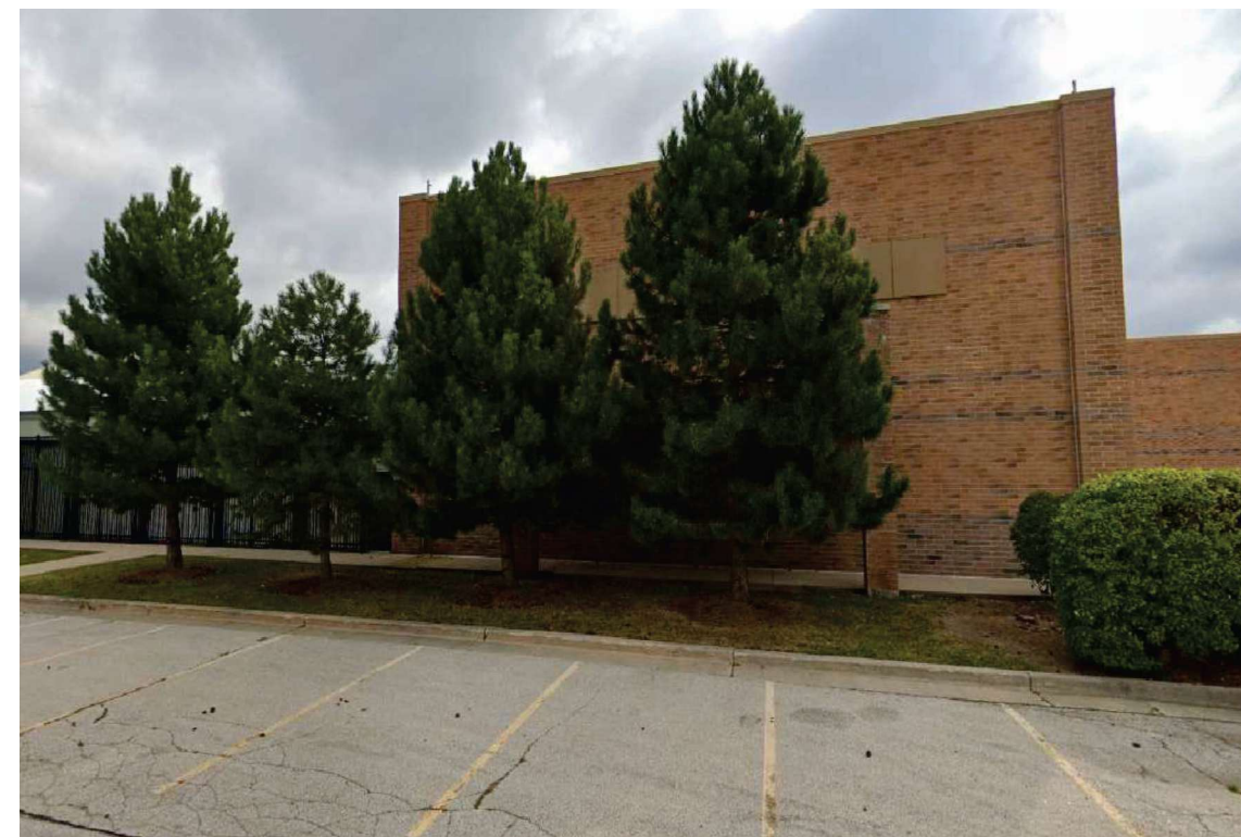
WEST SIDE OF EXISTING BUILDING
