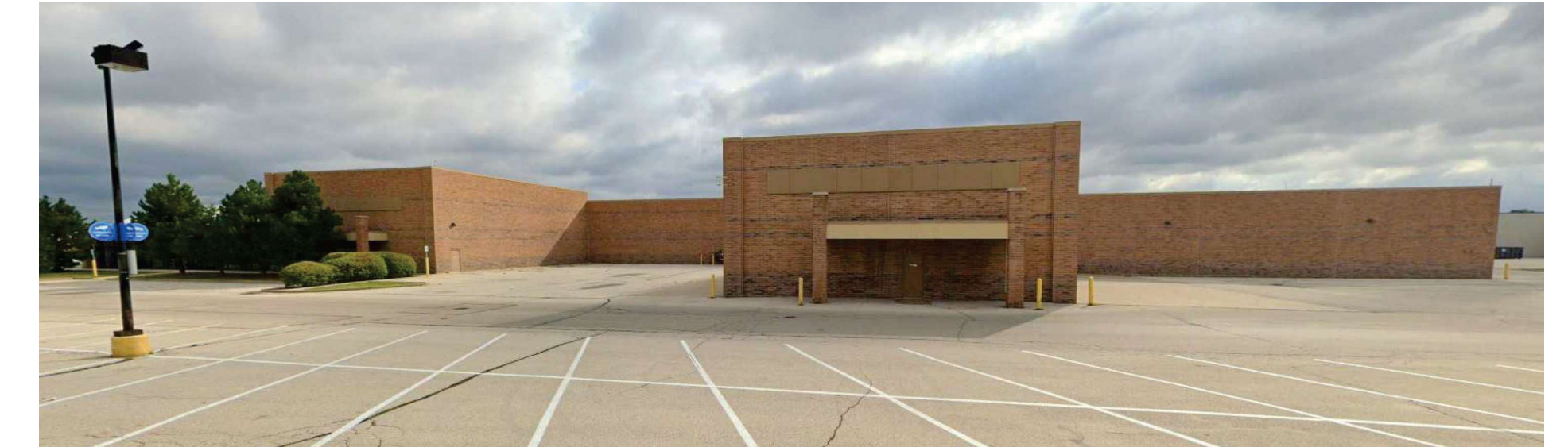
WEST SIDE OF EXISTING BUILDING
