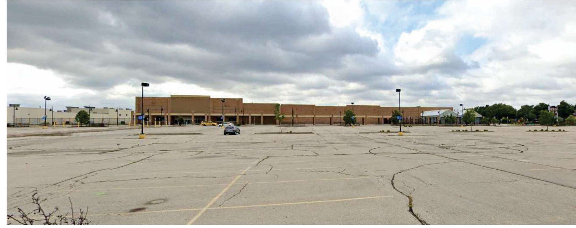
NORTH FACE OF EXISTING BUILDING
