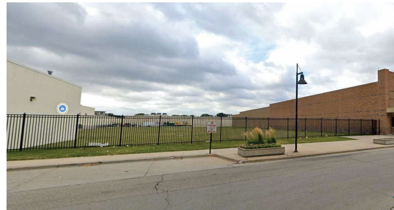
OPEN GREEN SPACE AT EAST SIDE OF BUILDING LOCATION OF FUTURE CITY OF MKE PARKING
