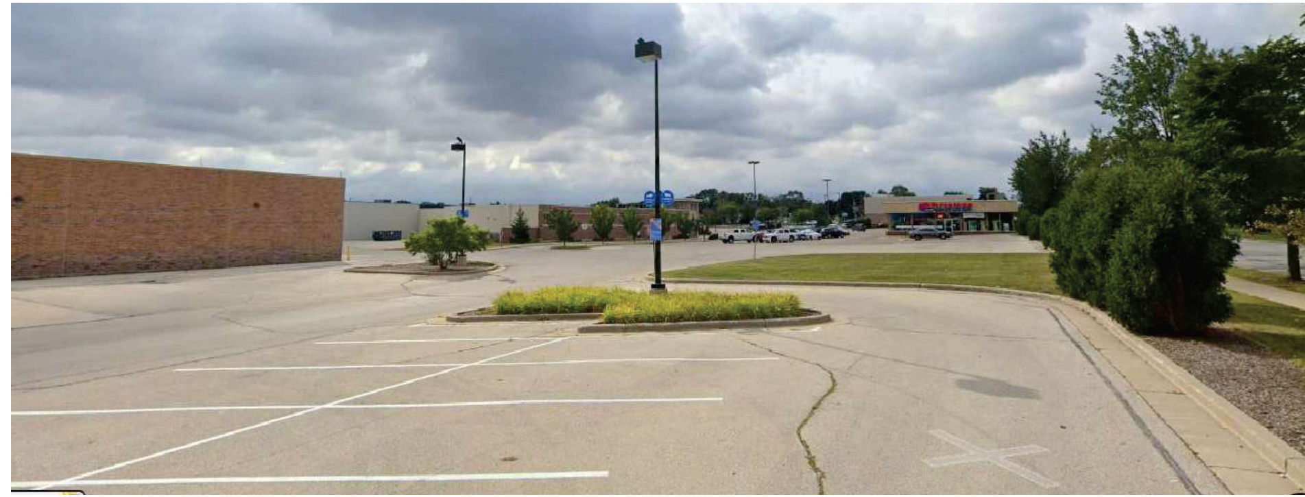
SOUTHWEST CORNER OF EXISTING BUILDING
