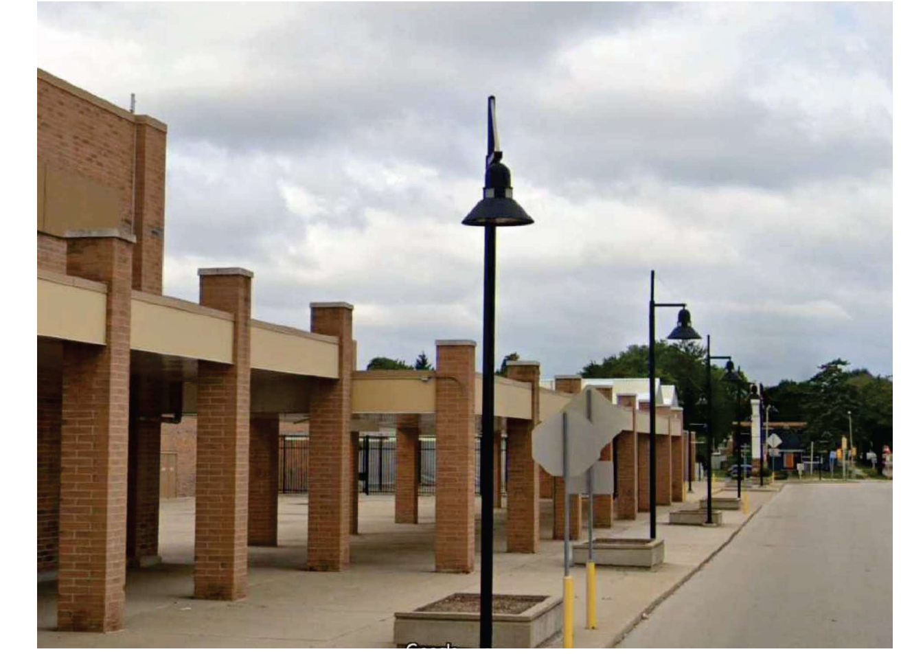
NORTH SIDE OF BUILDING LOOKING WEST
