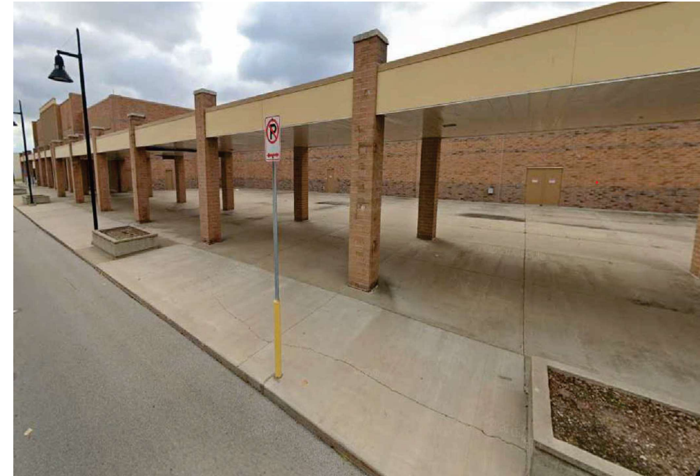
NORTH FACE OF BUILDING - COLONNADE
