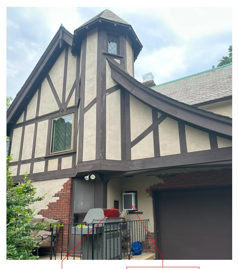
HISTORIC MILK DELIVERY DOOR REMAINS. AC UNIT TO BE REMOVED FROM WINDOW OPENING AND REPLACED WITH MARVIN ULTIMATE WINDOW. SEE NEXT PAGE FOR WINDOW SPEC.
