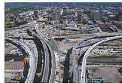
Marquette Interchange under construction
