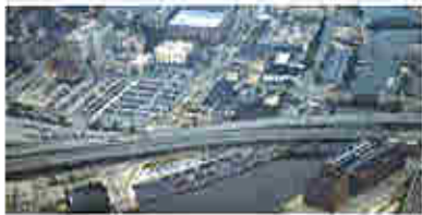
Park East Freeway before removal
