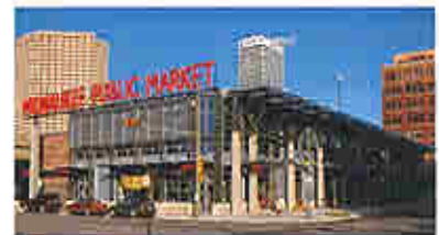
Milwaukee Public Market, N Water St and E. St Paul Ave.
