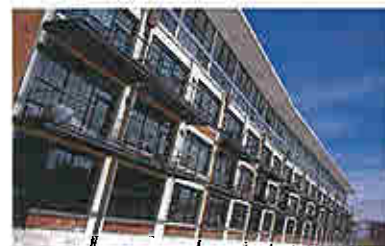
Marine Terminal Lofts, E. Erie St.
