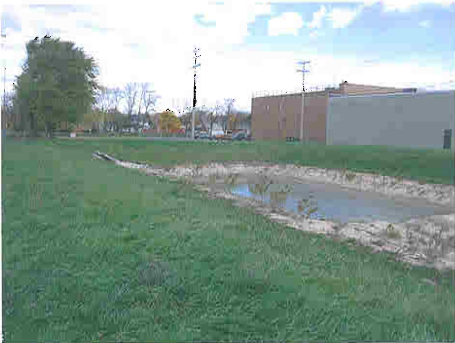
Figure 5: Overview of detention basin.
