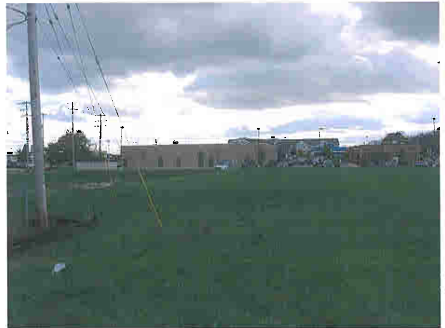
Figure 4: Detention basin located adjacent to the southeast corner of the site.
