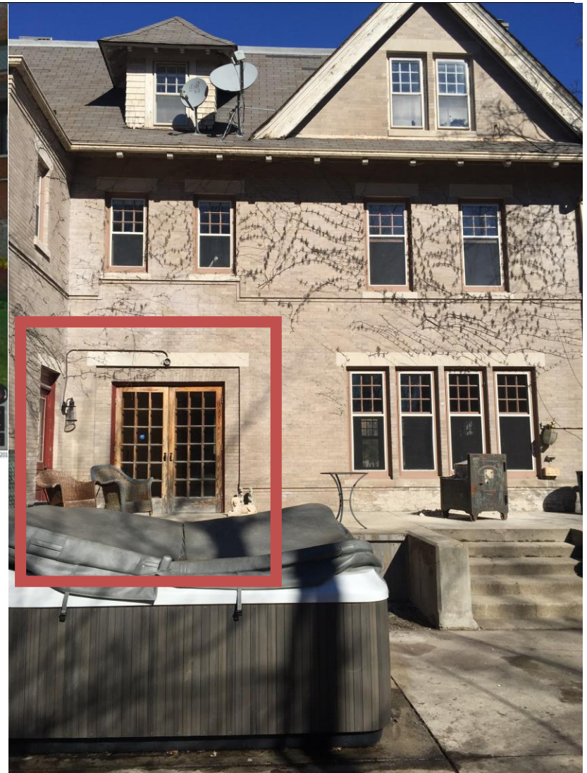
Rear view. All screen doors in this view to be replaced.
