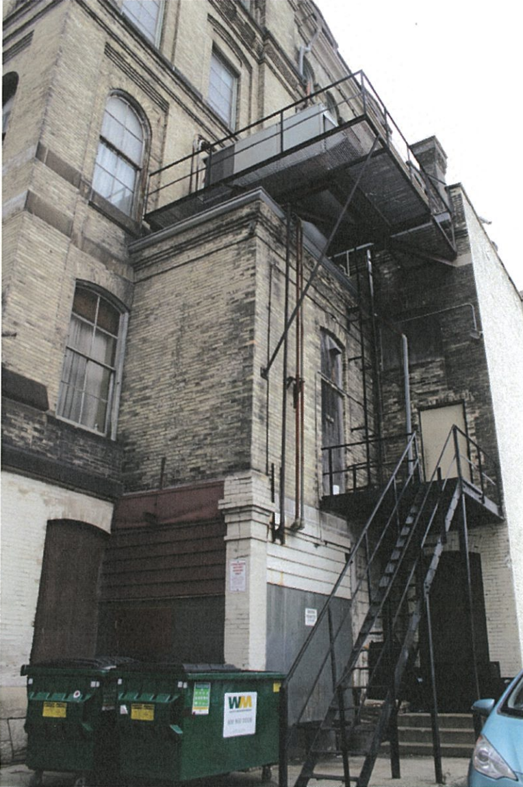
Photo No. 52: Looking northeast - showing southwest corner of building
