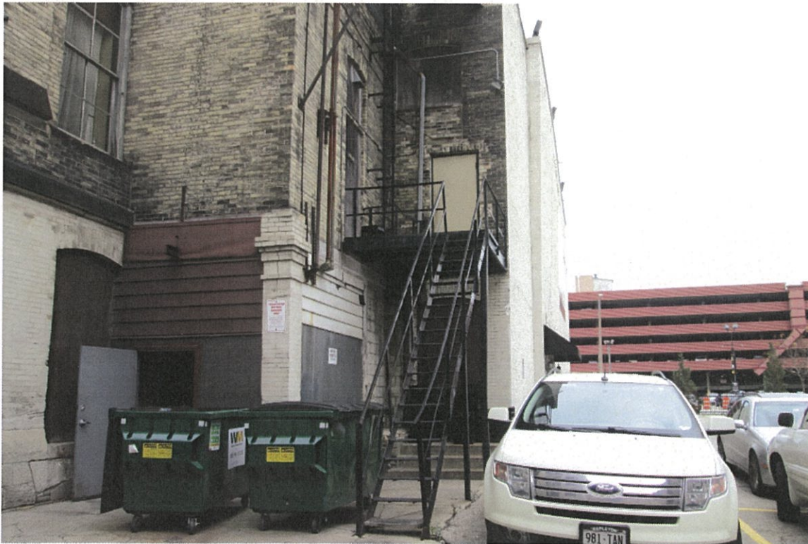
Photo No. 54: Looking east at southwest corner of building
