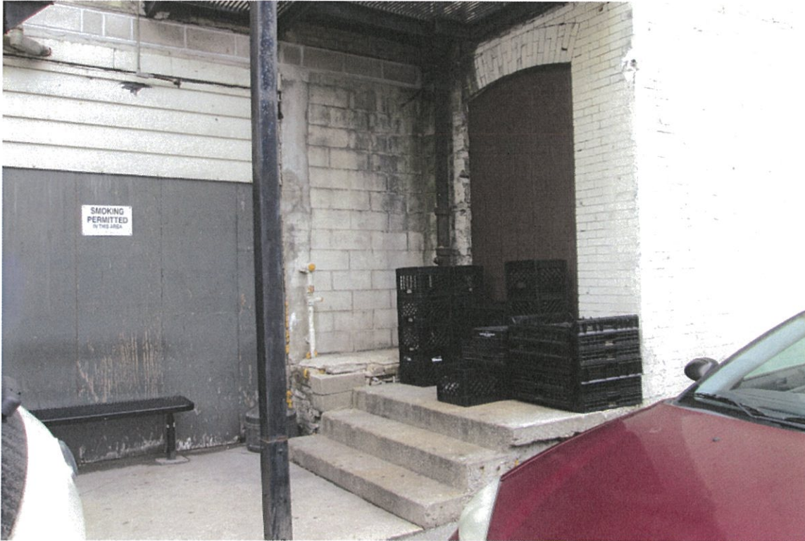
Photo No. 56: Looking north at lower level southwest corner of building
