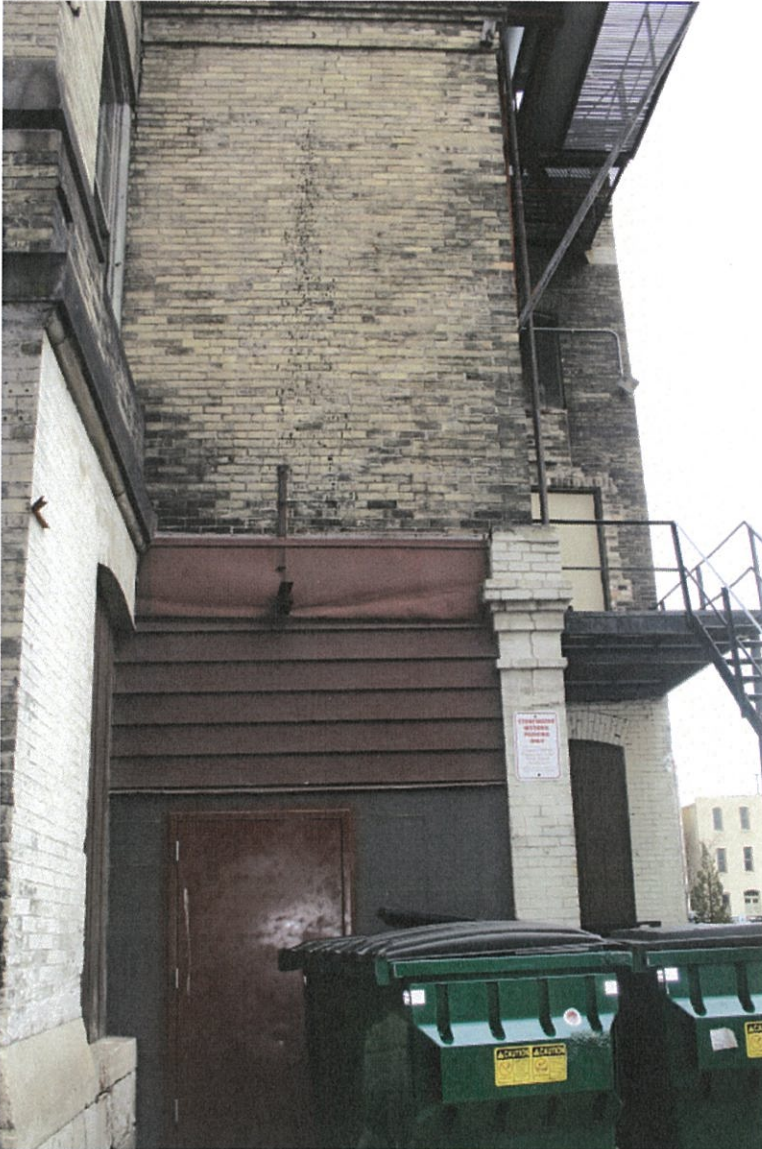
Photo No. 51: Southwest corner of building - location for new two-story addition
