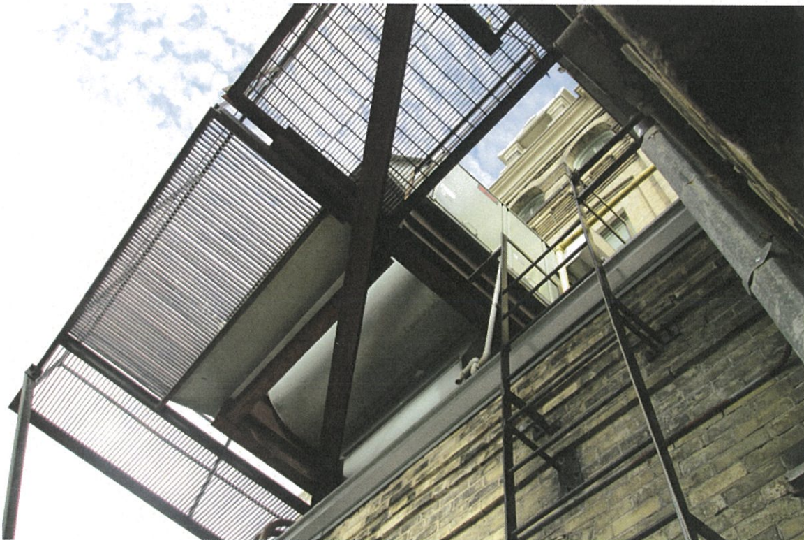
Photo No. 55: Looking up at steel platforms
