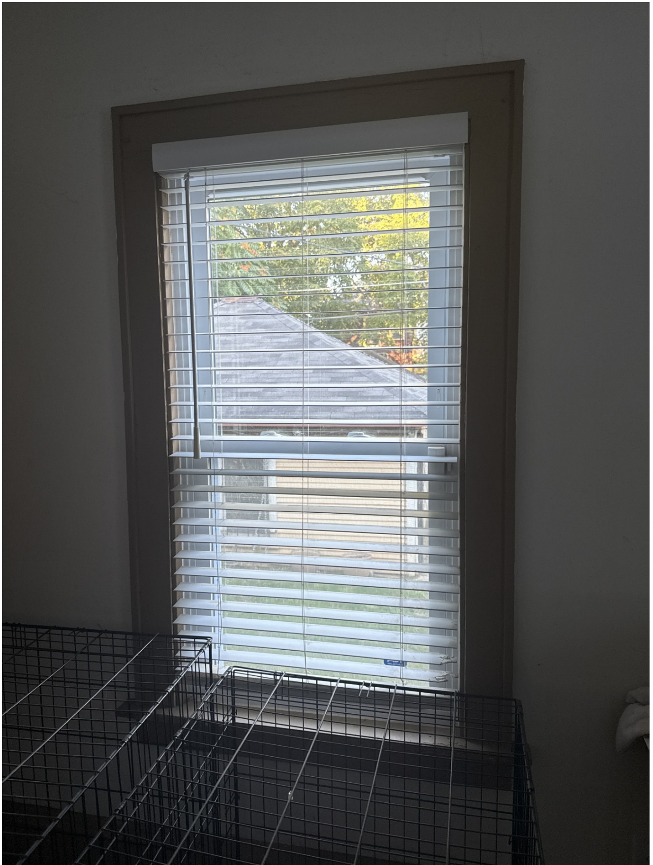
Second floor bedroom
