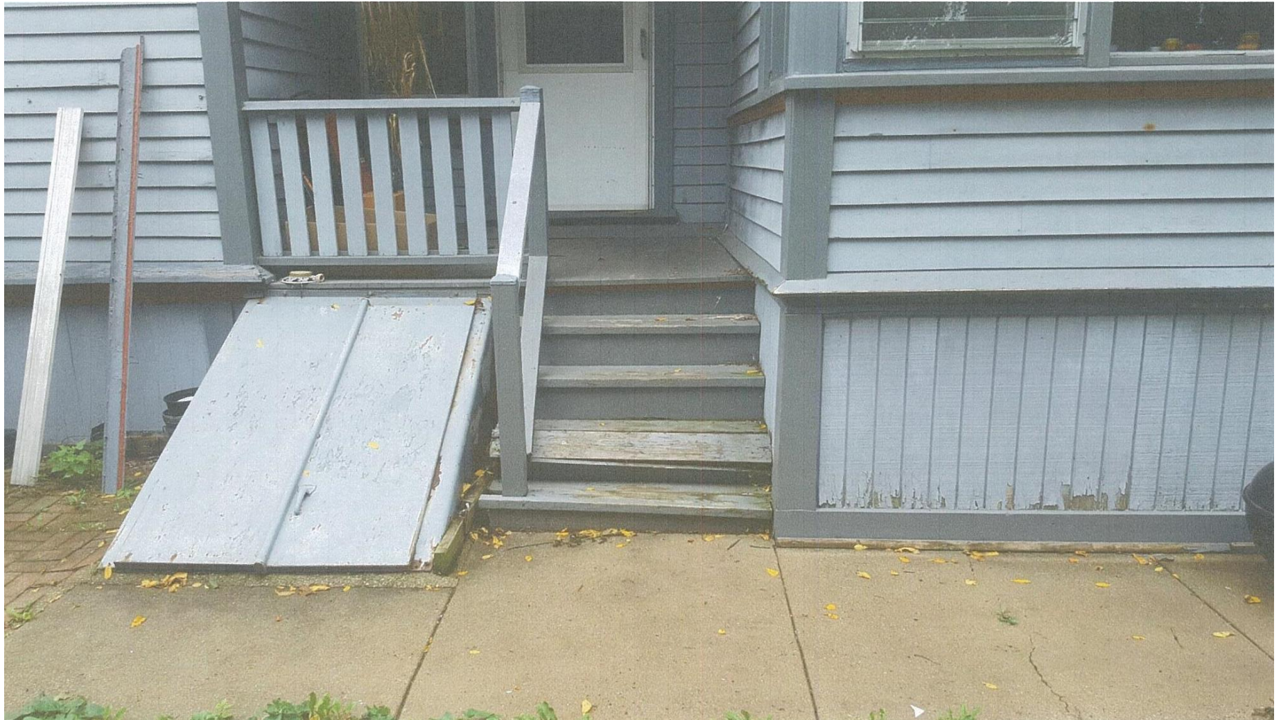
Back porch showing existing condition.
