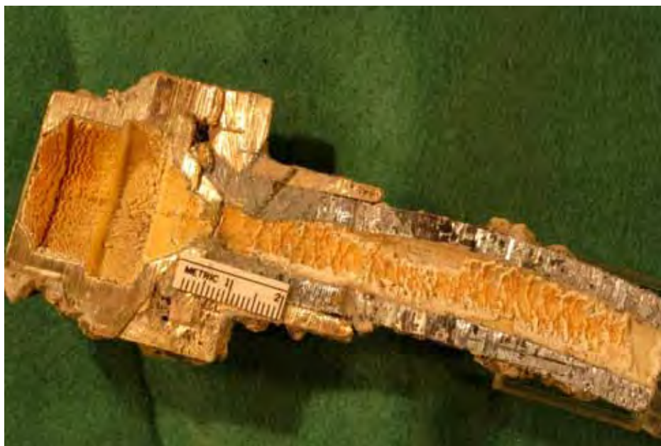
Figure F.70 Lead to Brass transition at Site T-4. The scale comprises a thick, white lower layer and a thin brown-red upper layer on both lead and brass components.
