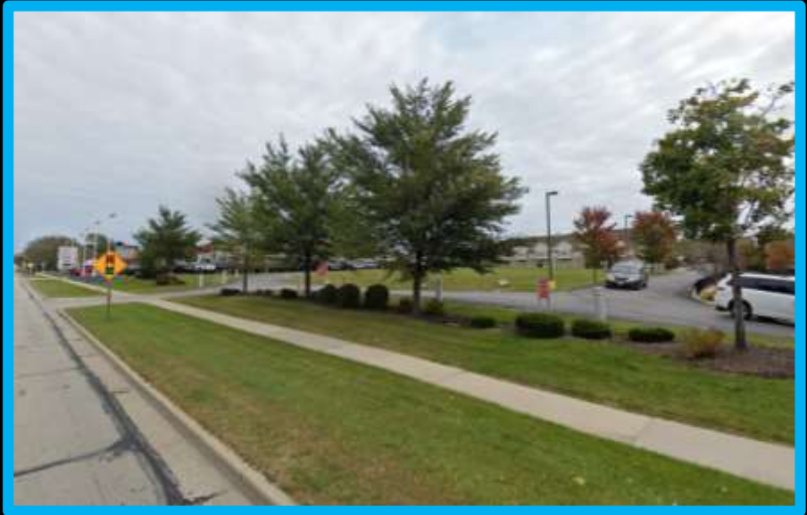
View from South 27 th Street looking north-east
