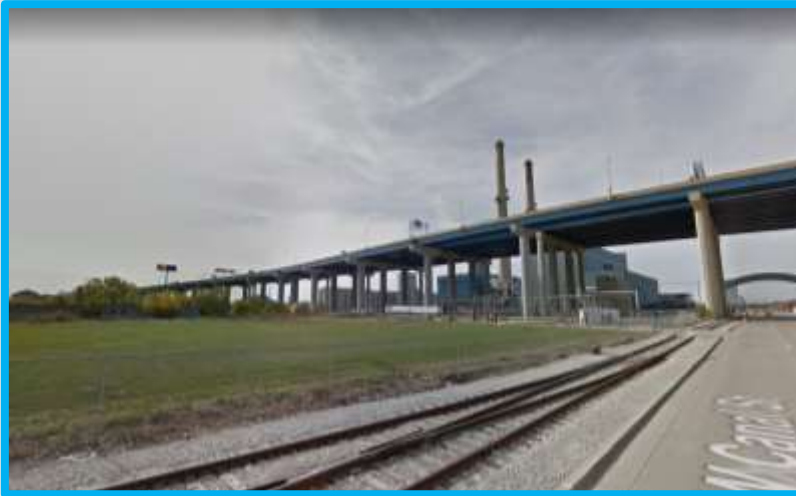
View from W Canal St looking southwest
