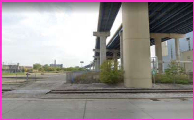
View from W Canal St looking south
