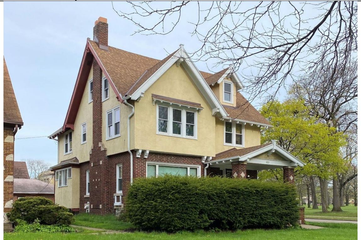
Current view looking NW.
