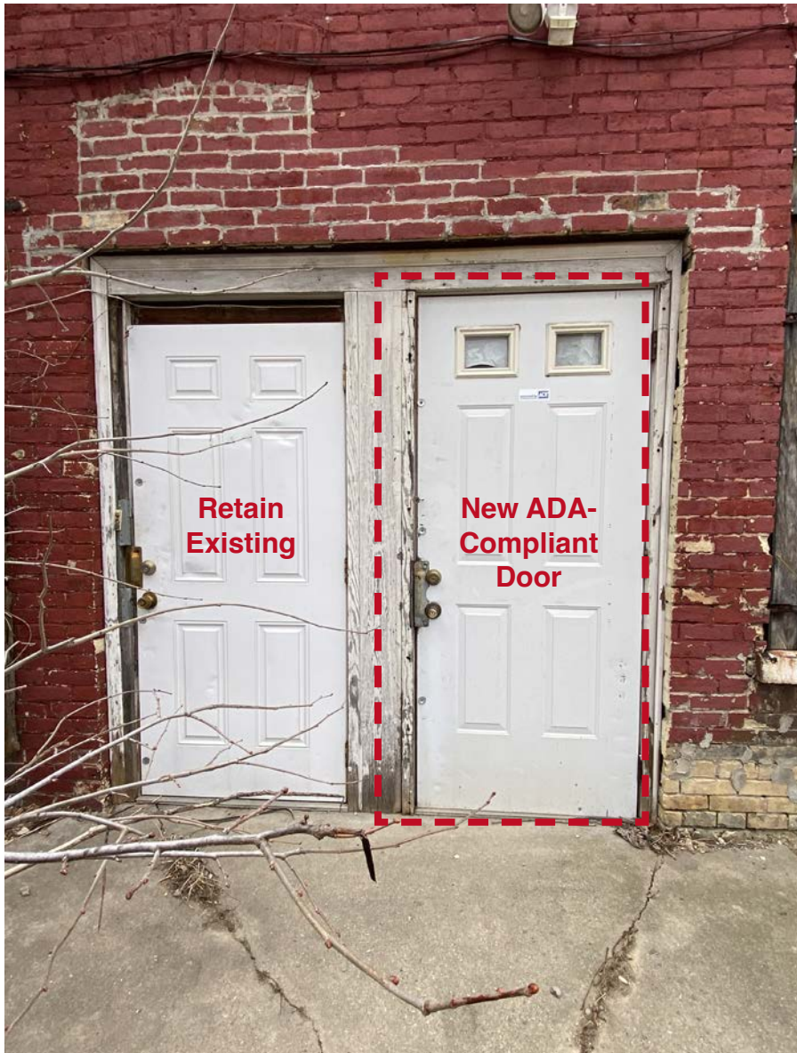
IMAGE 16: Detail view of west elevation doors. The door on the left will be retained and the opening reconfigured to fit more tightly. The door on the right will be replaced with an ADA compliant door as described in the Scope Narrative. Trim around the doors within the masonry opening will be reconfigured and refinished to match the doors and to better address voids. No work is anticipated at the steel lintel.
