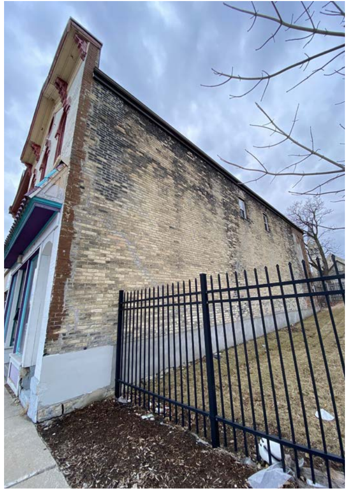
IMAGE 15: North elevation; here work is limited to masonry repairs and flashing at windows as described in the Scope Narrative.
