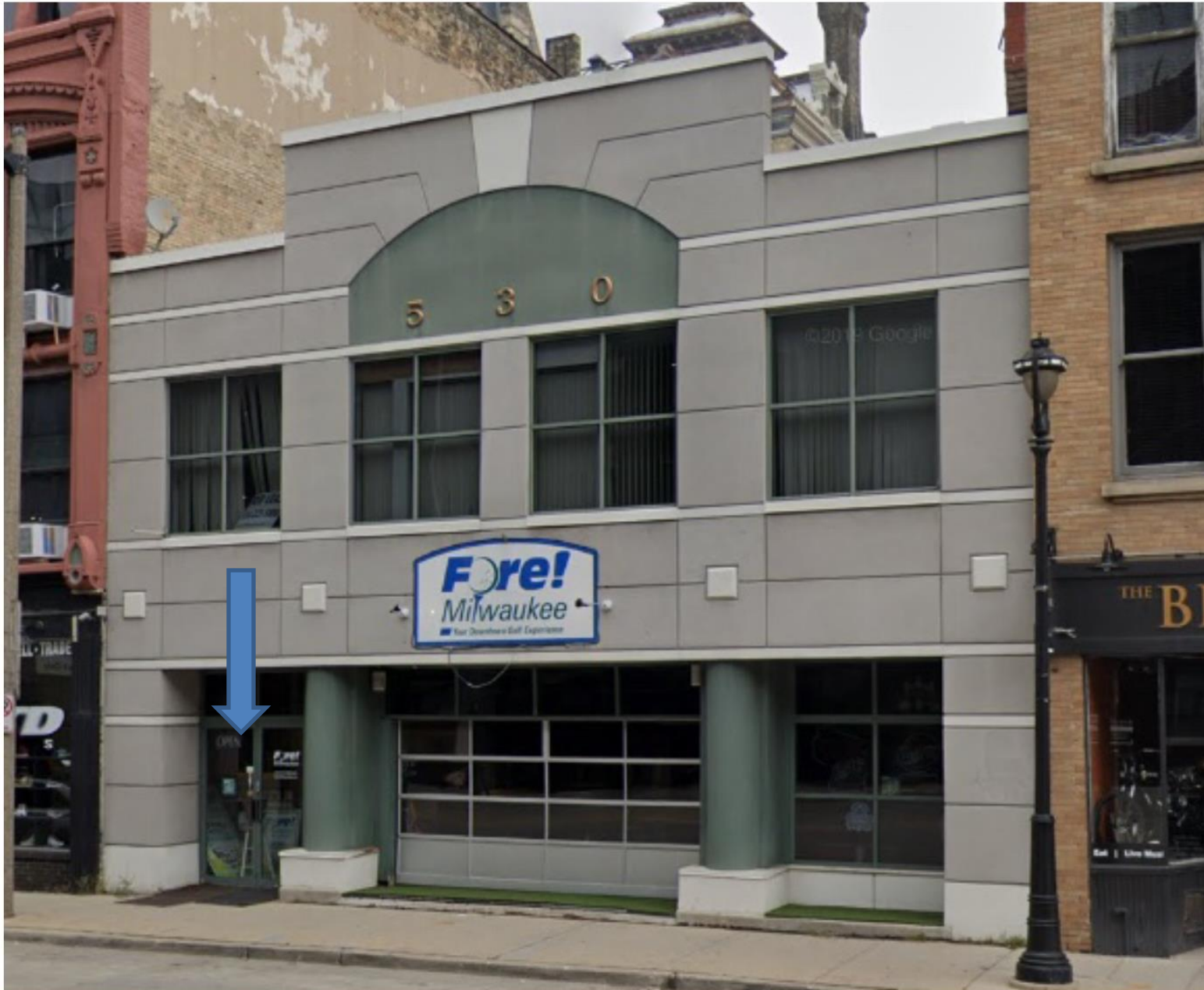
Current conditions with subject door identified.
