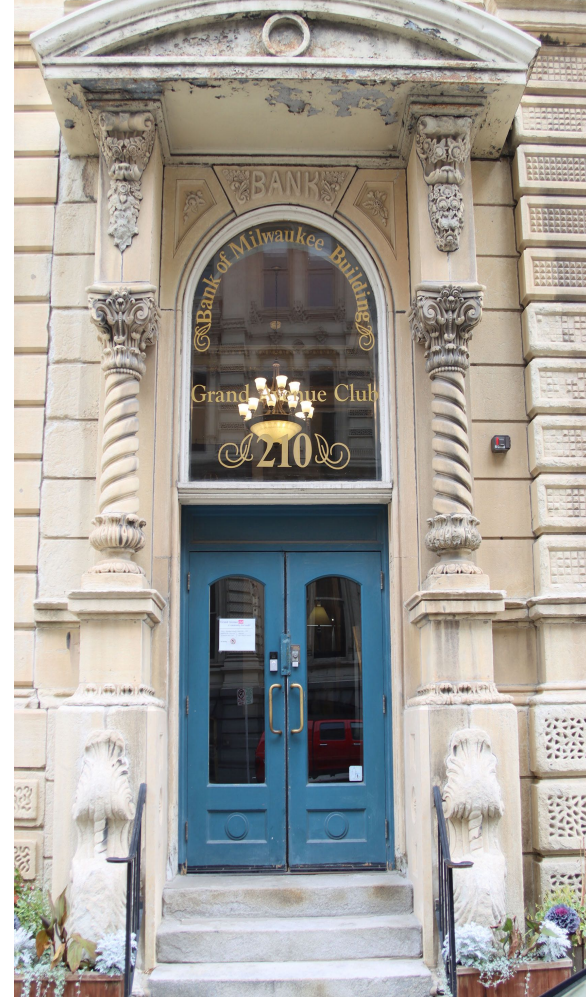
EXISTING ENTRY LOCATION (SOUTH ELEVATION)
