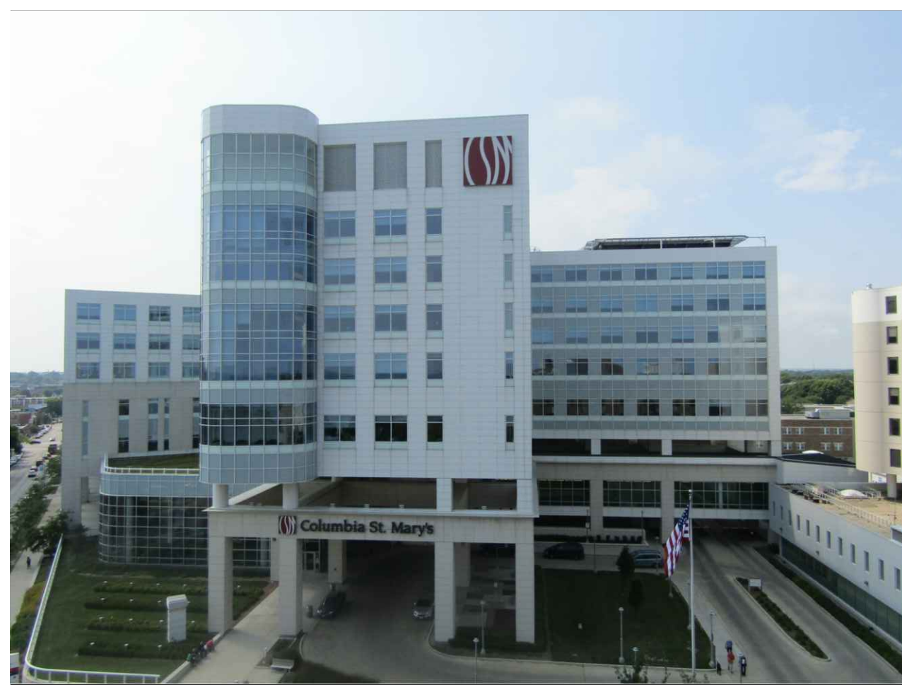
OVERALL VIEW OF EAST ELEVATION/FRONT ENTRANCE OF THE MAIN HOSPITAL
