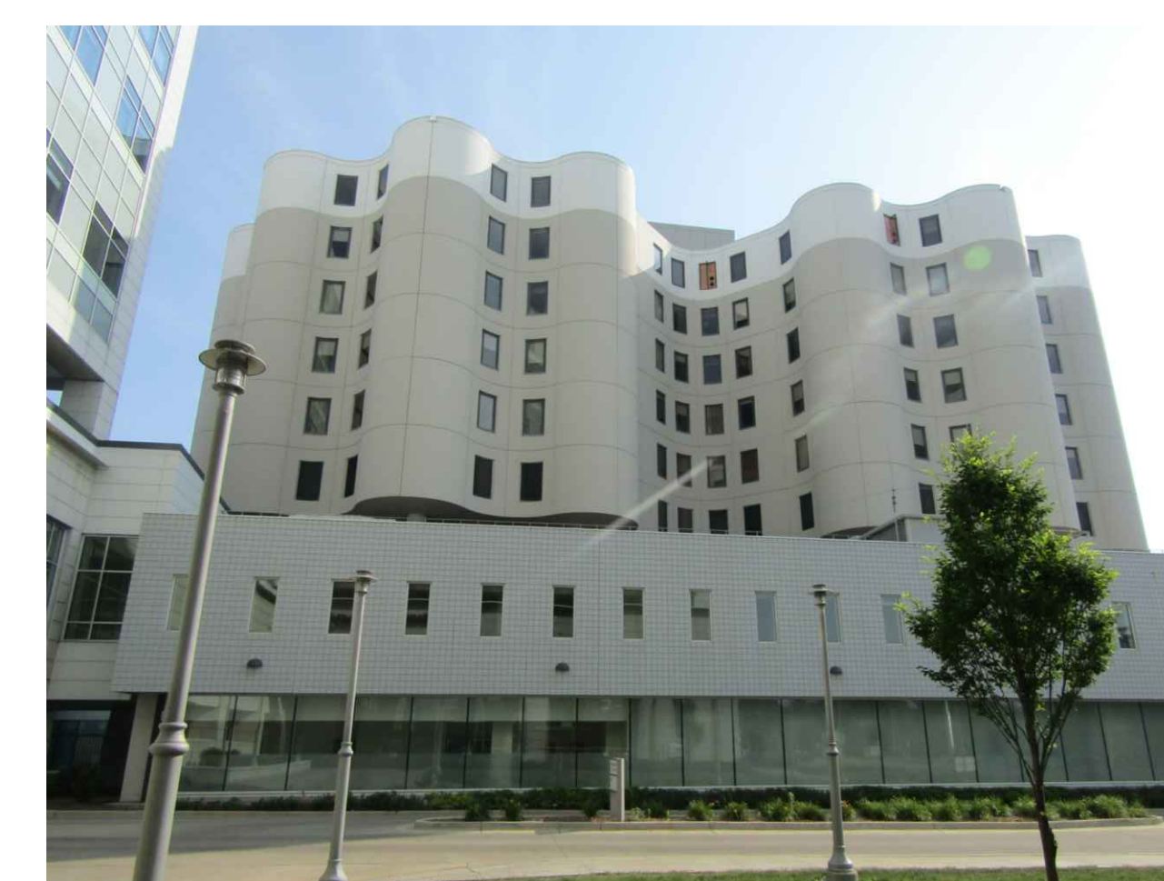
OVERALL VIEW OF SOUTH ELEVATION WOMEN'S HOSPITAL BUILDING
