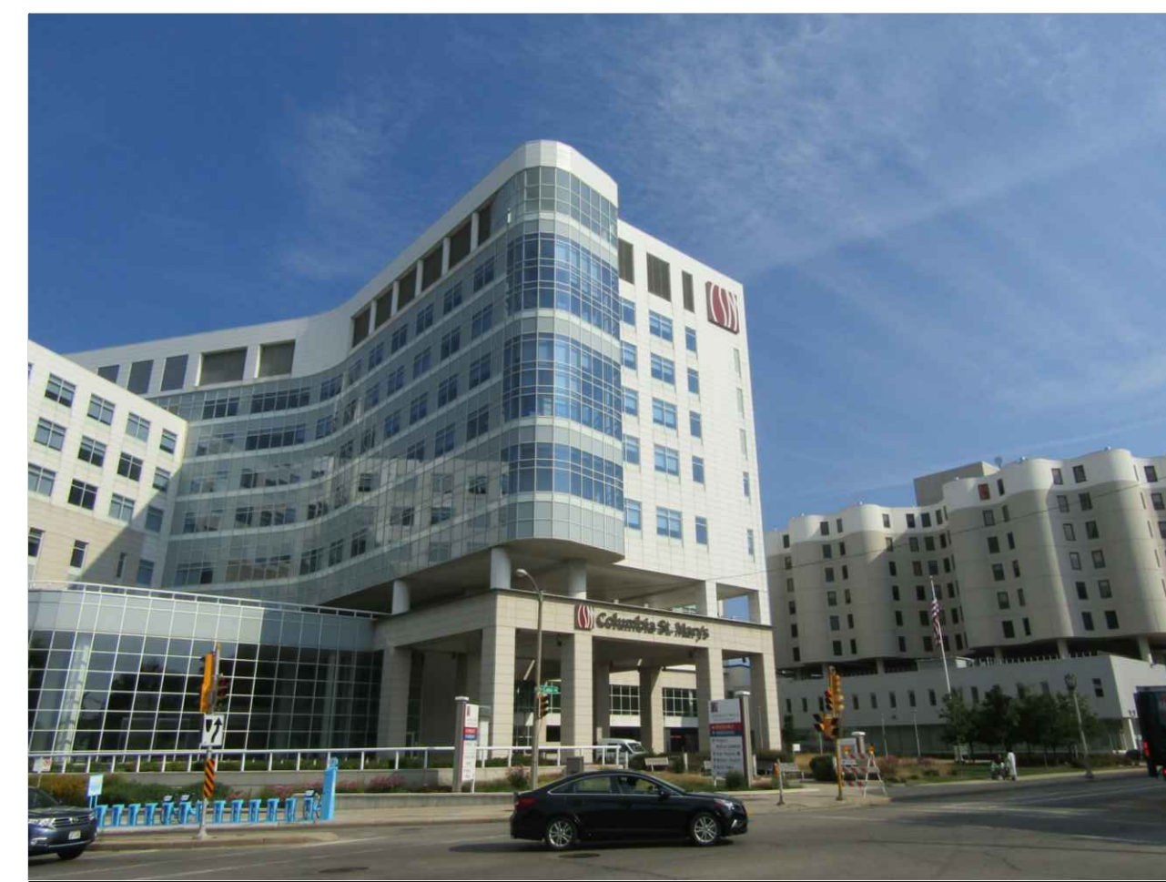
OVERALL VIEW OF SOUTH AND EAST ELEVATIONS OF MAIN HOSPITAL
