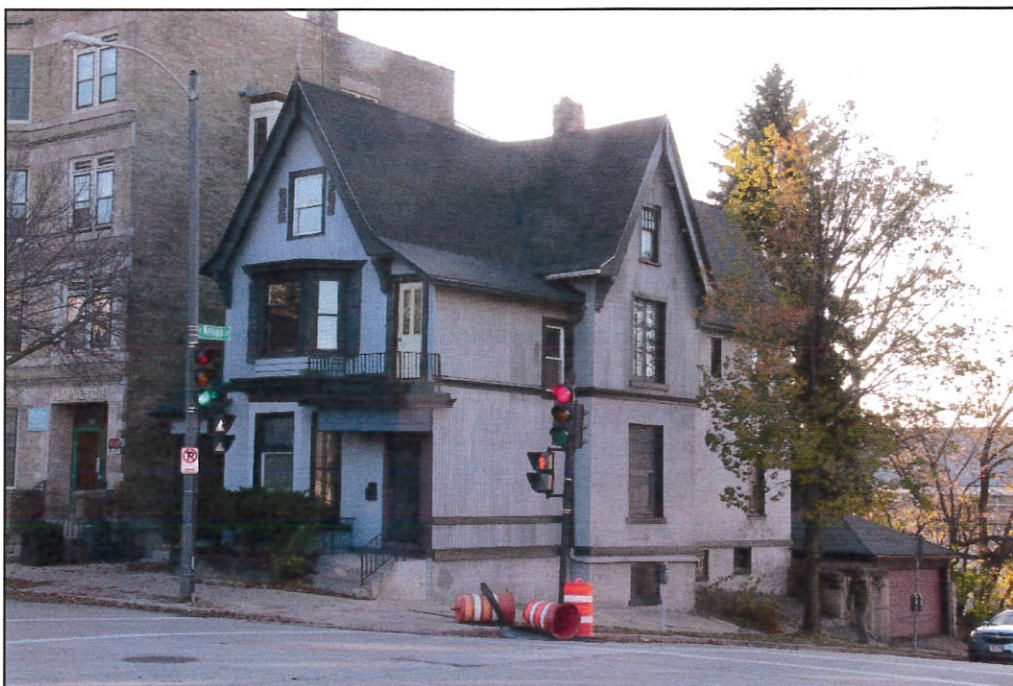
Figure 1: 1245 N. Milwaukee Street. View to southwest.
