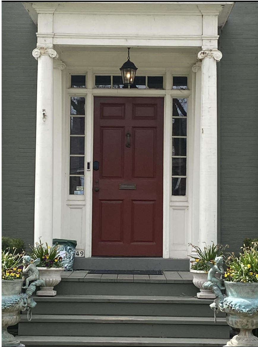
Existing porch columns
