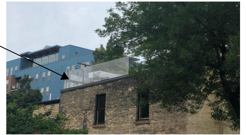
Facing North East looking at the west face
