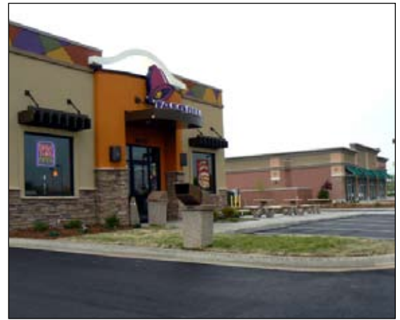
Outlot developments at Granville Station.
