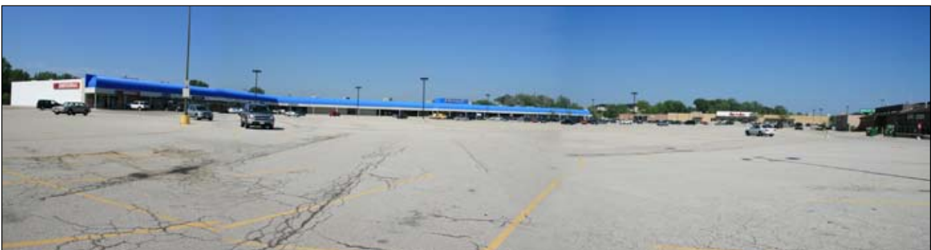
Existing conditions at Timmerman Plaza.
