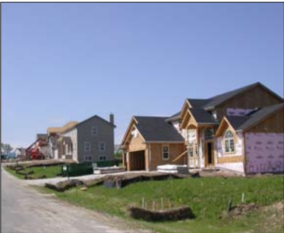
Construction of single-family homes off of County Line Rd.
