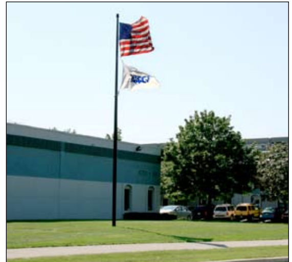
Direct Supply is a growing campus on Industrial Road
