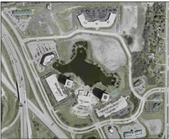
An aerial image of the Park Place office cluster, located east of US 41/45.
