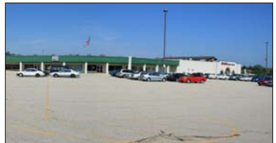
Existing conditions of the strip mall north of Granville Station.
