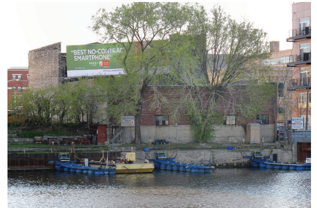
00.4 existing street NORTH / REAR facade
