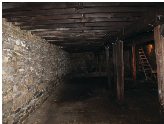
09.3 east bay EAST view
