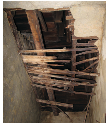
01.7 east bay CEILING
