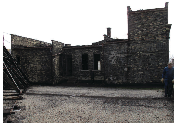
08.1 J.L. Burnham building rear facade SOUTH view
