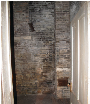
04.1 garage room south view at entry
