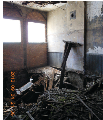
02.6 center bay SOUTHWEST view
