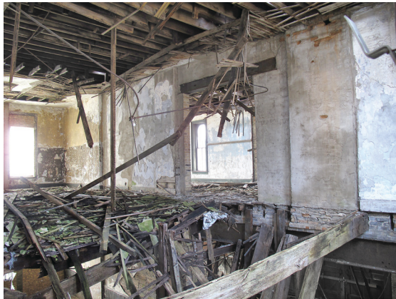
06.1 center bay WEST view from garage roof
