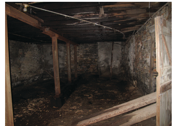
11.4 west bay SOUTH view
