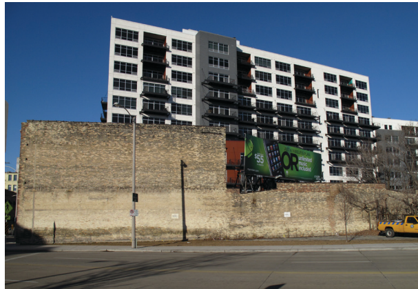
00.1 existing street EAST facade
