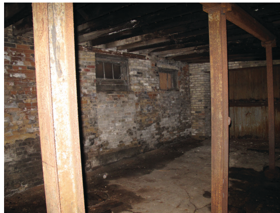
11.1 west bay WEST view
