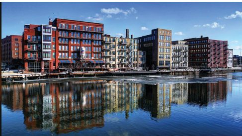
Milwaukee Ale House
