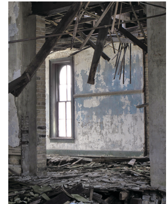
07.2 west bay WEST view
