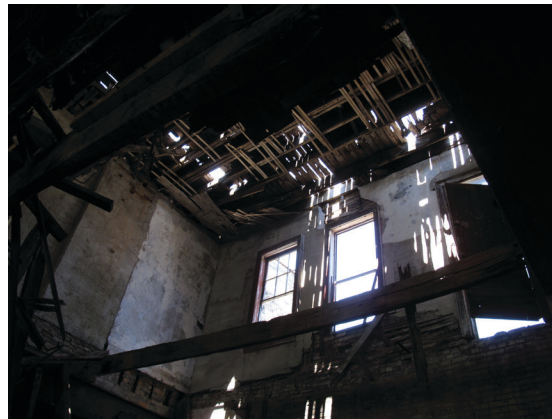
06.5 center bay CEILING from below
