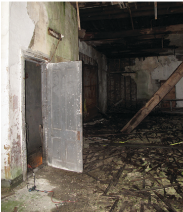
01.1 east bay WEST view at stair entry
