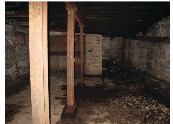
11.2 west bay NORTH view
