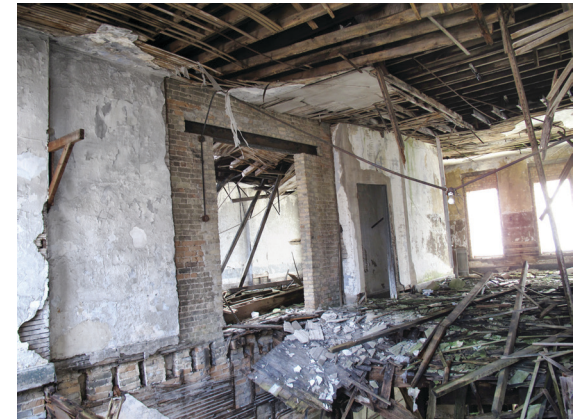
06.3 center bay EAST view from garage roof
