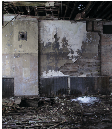
02.1 center bay WEST view from stair hall
