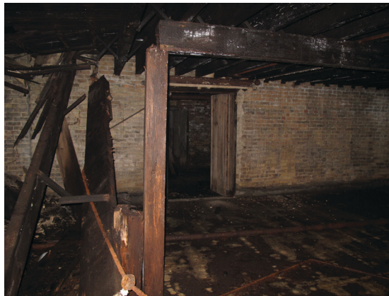
10.1 center bay WEST view
