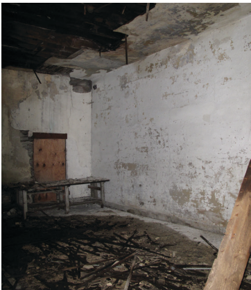
01.5 east bay EAST view
