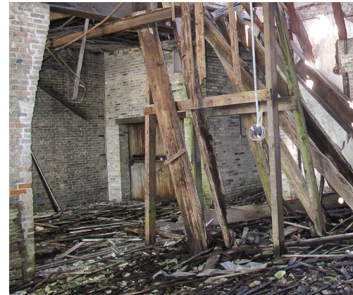
03.2 west bay NORTHWEST view at I-beam opening
