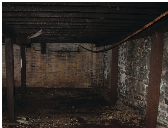
10.3 center bay SOUTHEAST view
