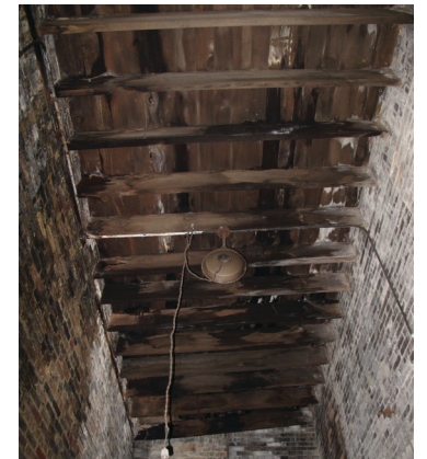
04.3 garage room CEILING
