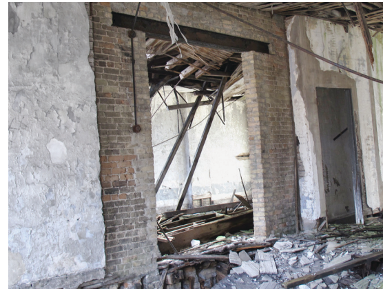
07.1 east bay EAST view
