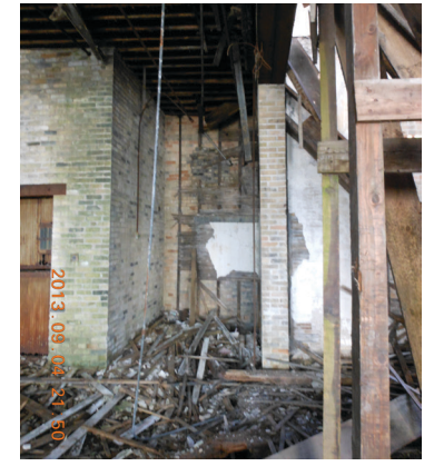
03.3 west bay NORTH view
