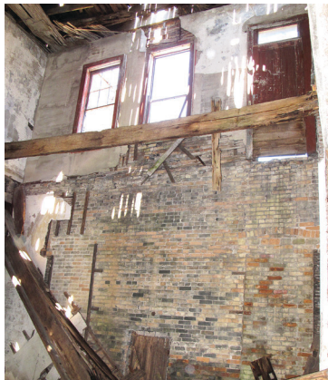
06.4 center bay NORTH view from below
