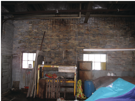
05.2 garage section NORTH view
