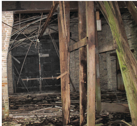
03.1 west bay WEST view from stair hall
