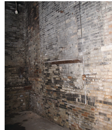
04.3 garage room SOUTHEAST view
