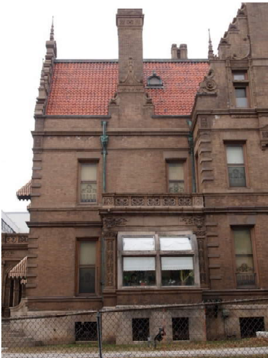
East Elevation Chimney
