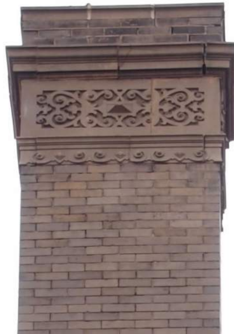
East Elevation Chimney Closeup
