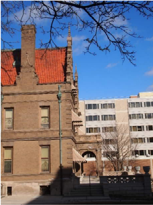
West Elevation Chimney
