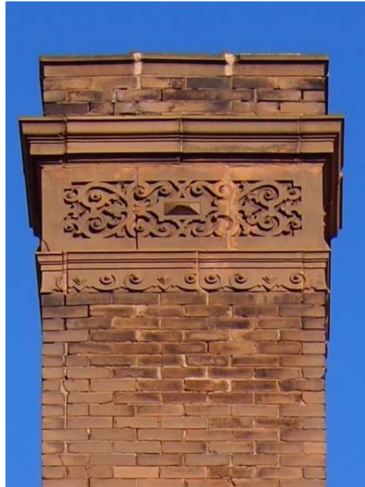
West Elevation Chimney Closeup
