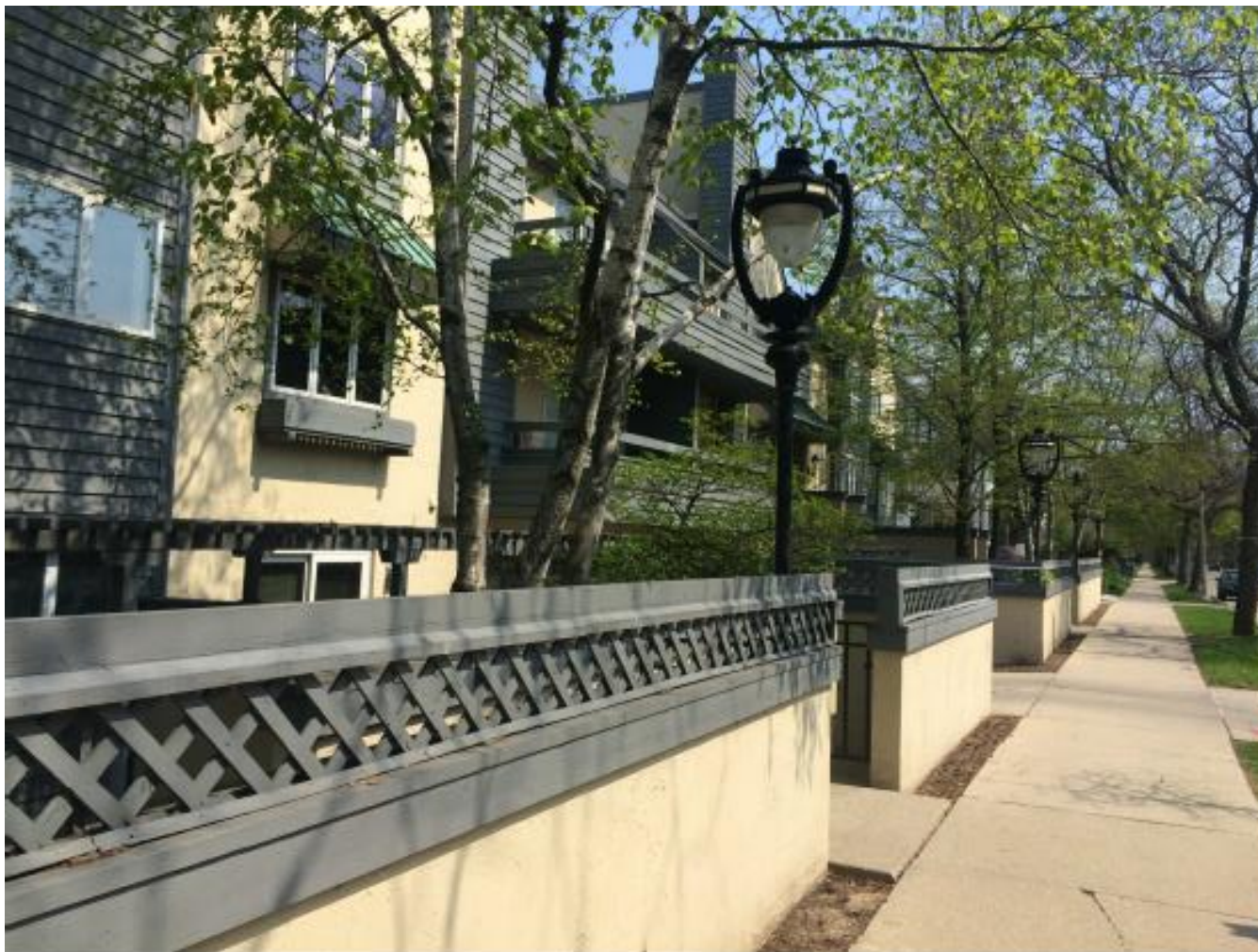
Pedestrian View traveling north - showing half wall to be renovated
