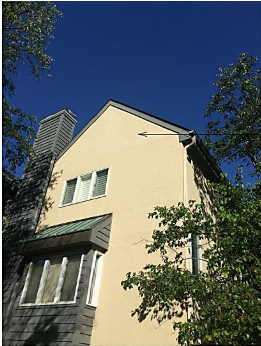
Exterior Facade - showing typical "telegraphing" of sheathing through EIFS finish
