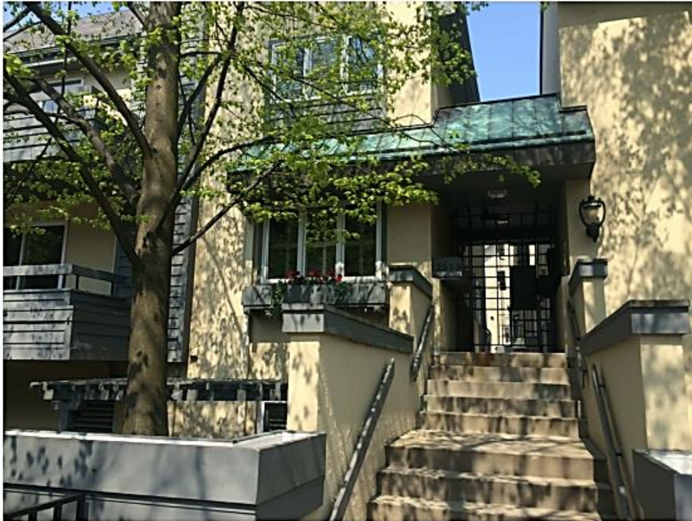
Existing entry gate area to be renovated
