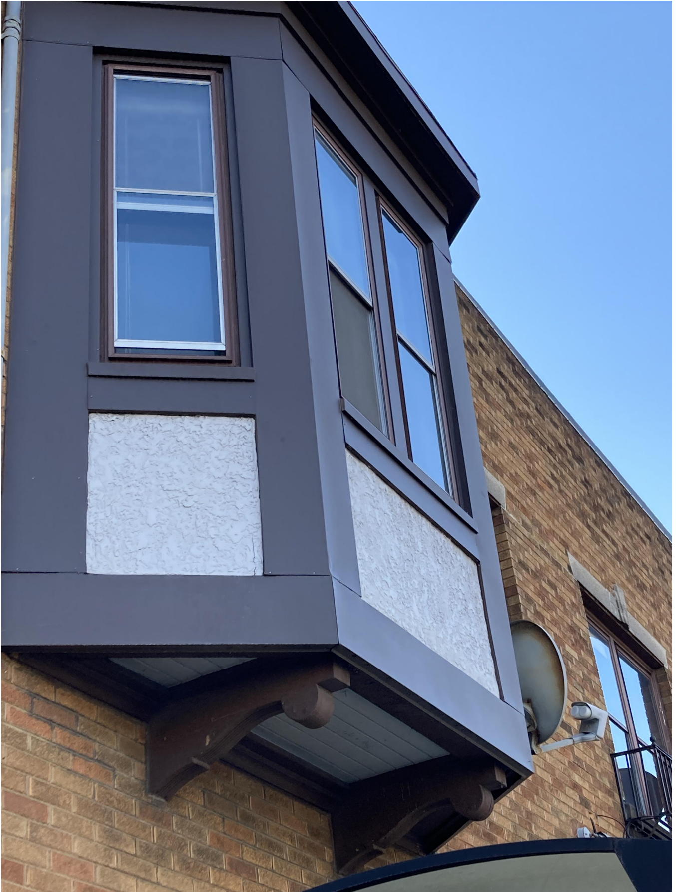
Existing textured panels on 2nd story bay window facing Layton Blvd.
