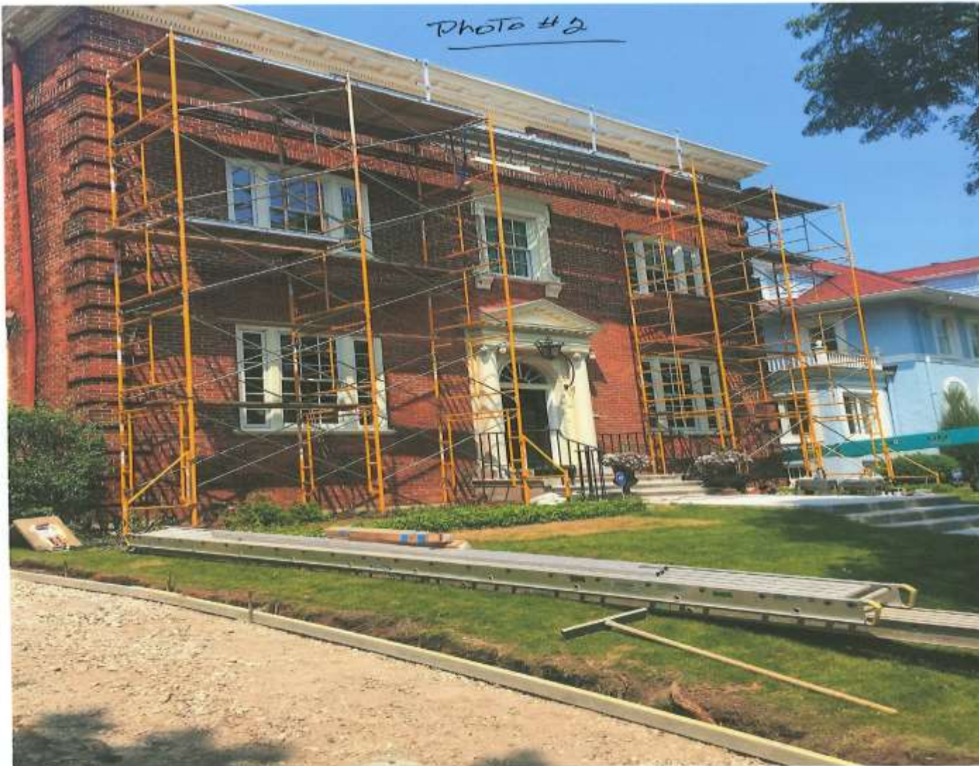
Photo showing work in progress and bushes removed.
