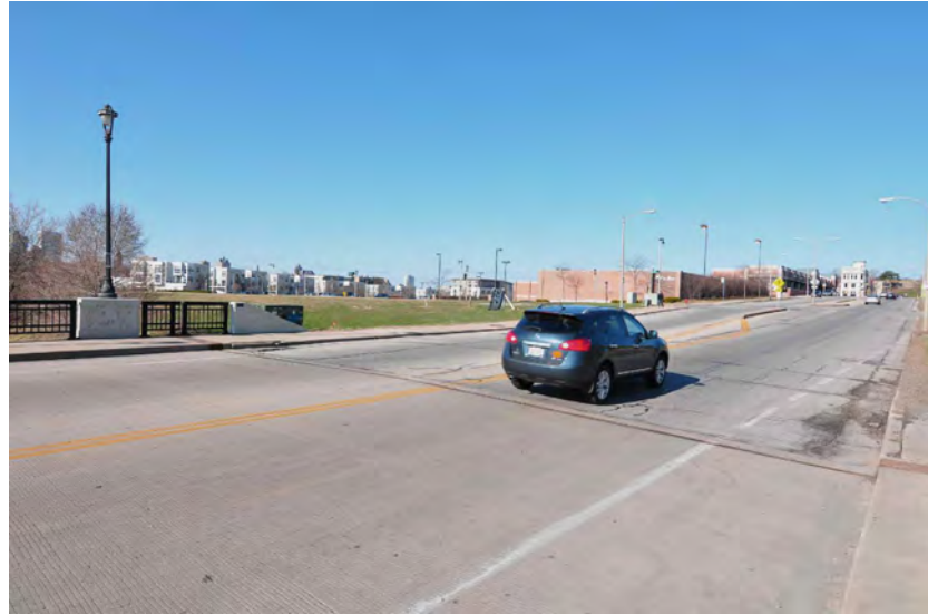
SITE VIEW 01: Looking west along North Avenue from North Avenue bridge
