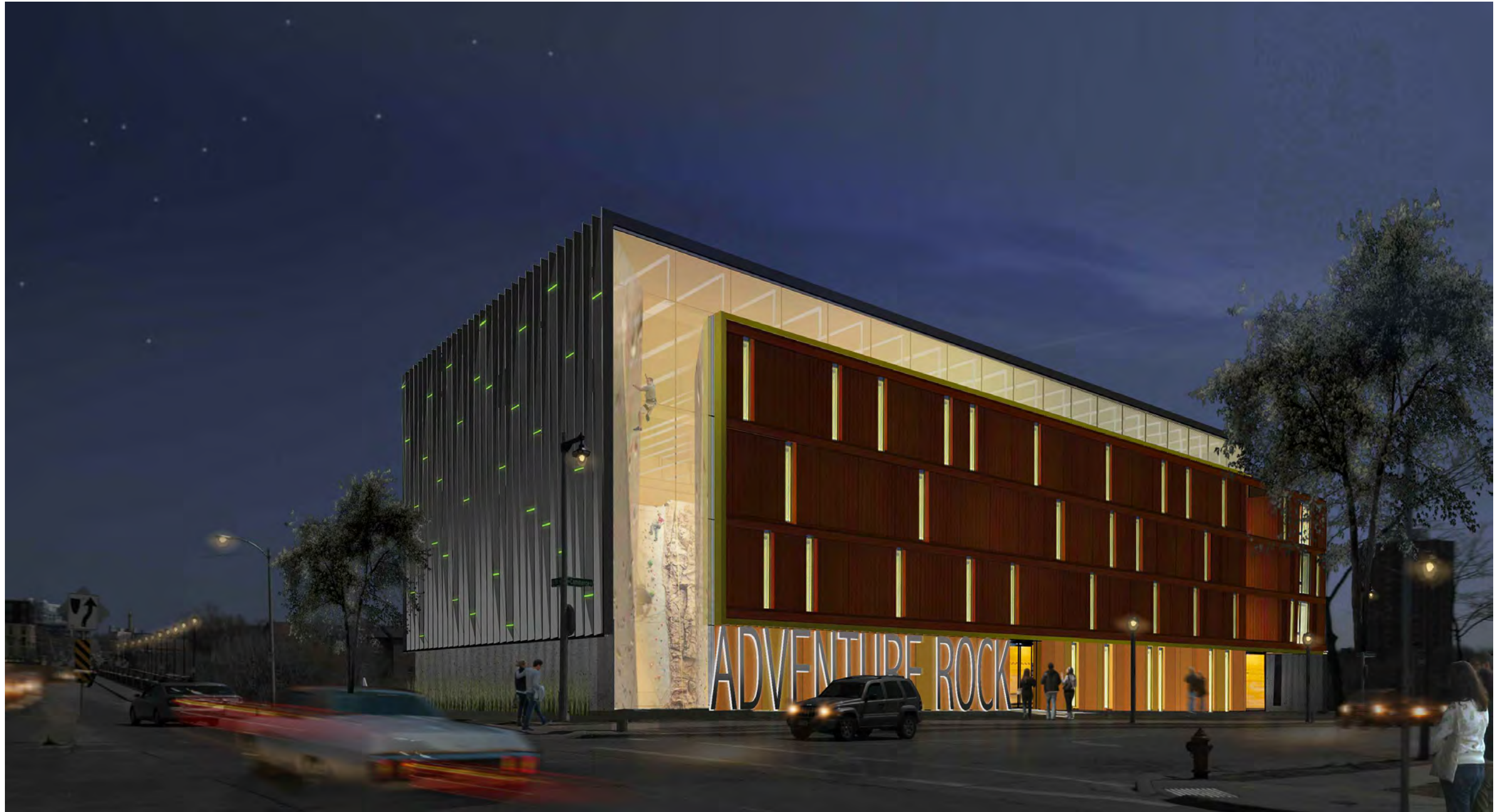
VIEW FROM EAST NORTH AVENUE
