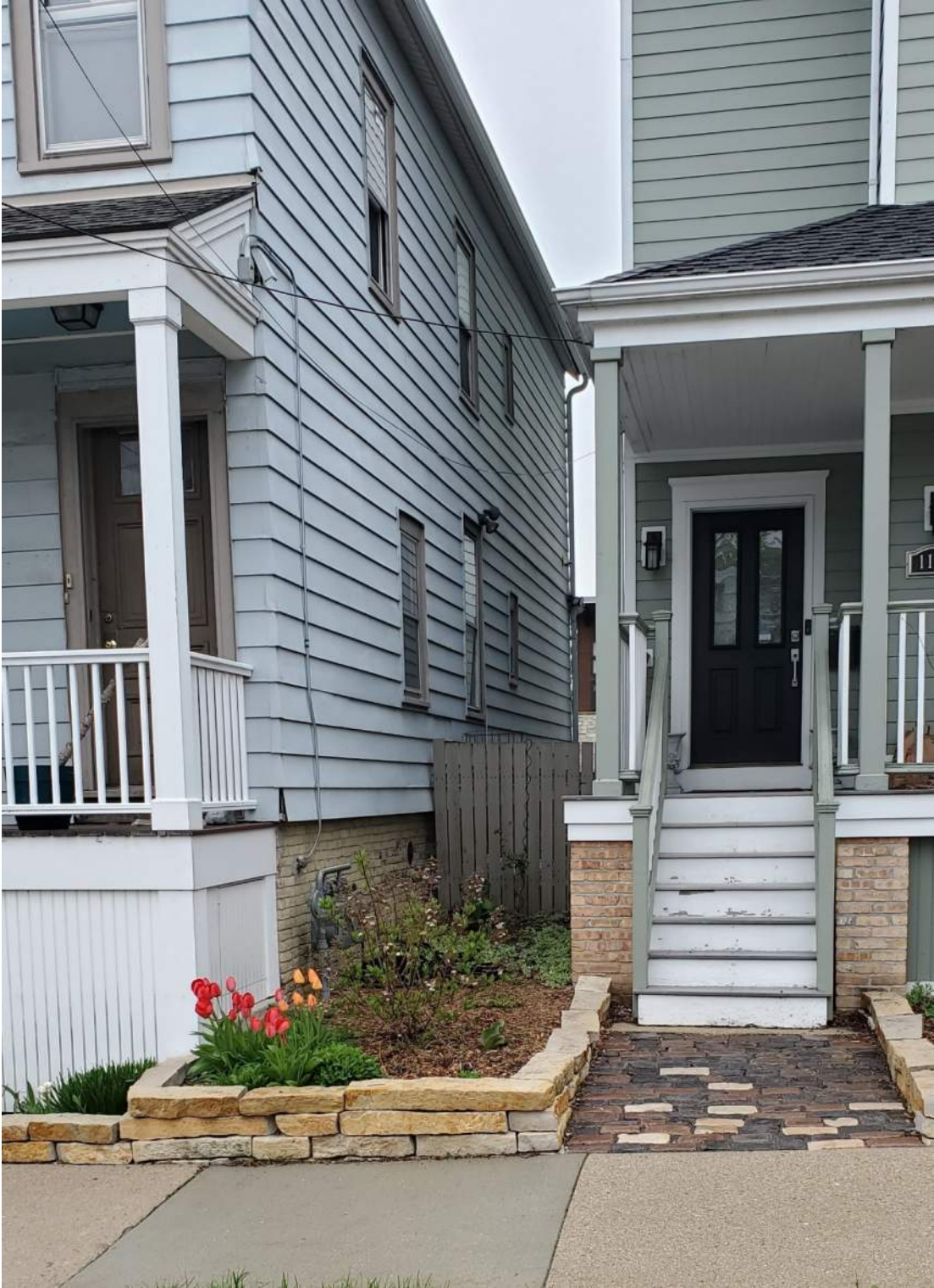
East Elevation looking north
