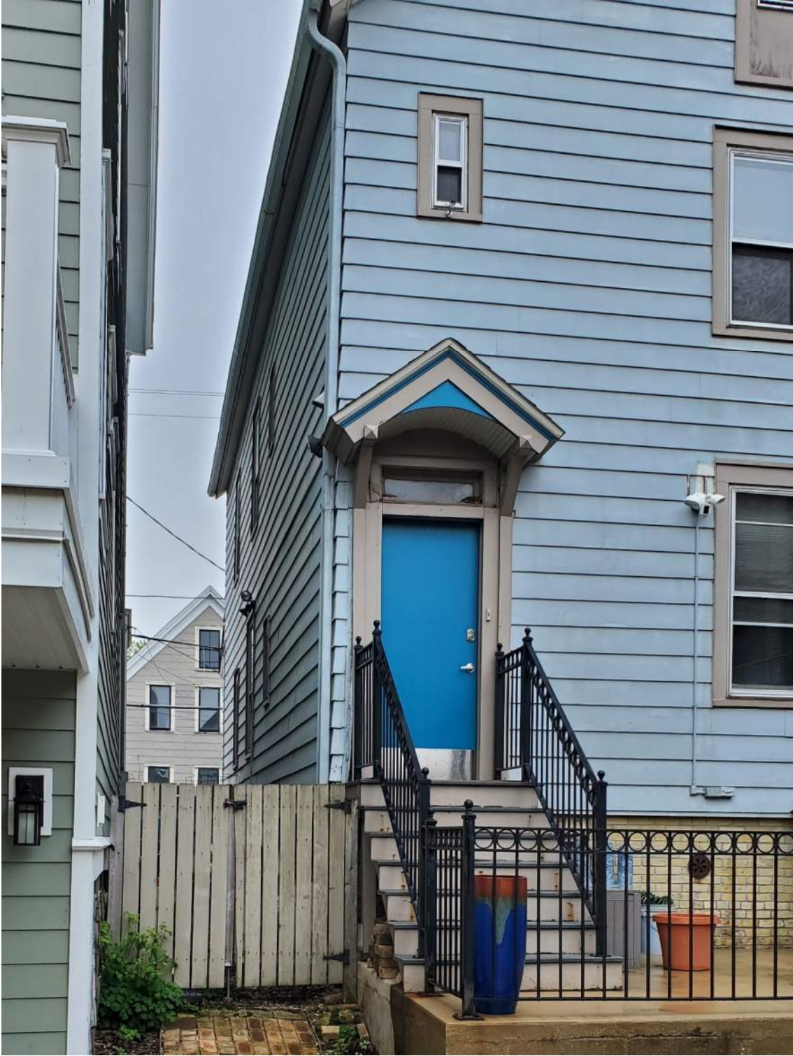
East Elevation Looking South
