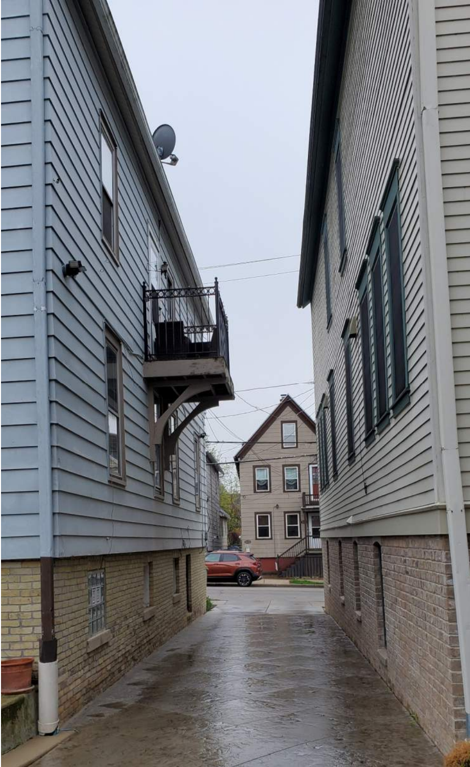
West Elevation Looking South
