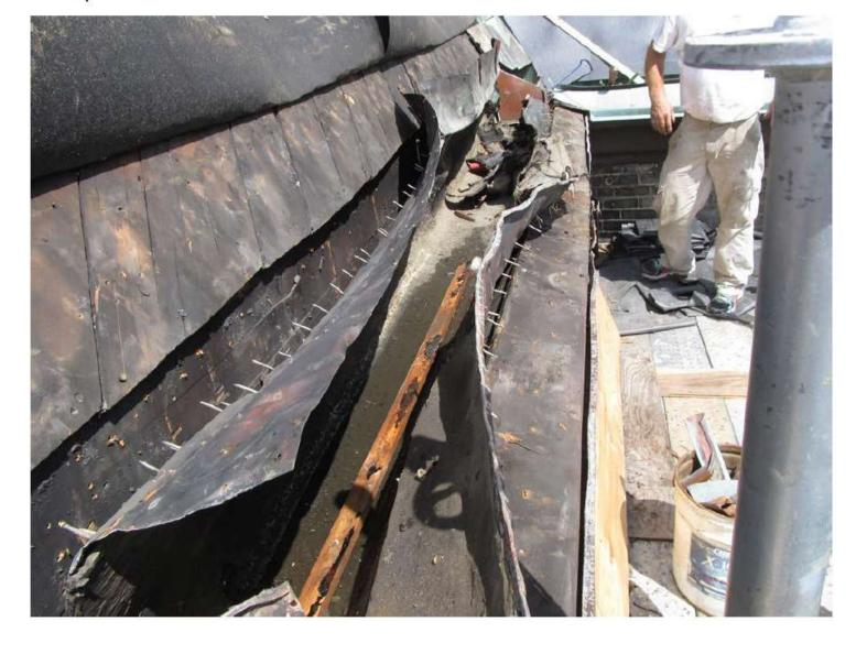
Photo 3 shows the new 20 ounce copper gutter liner set to the original cornice and the slate roof.
