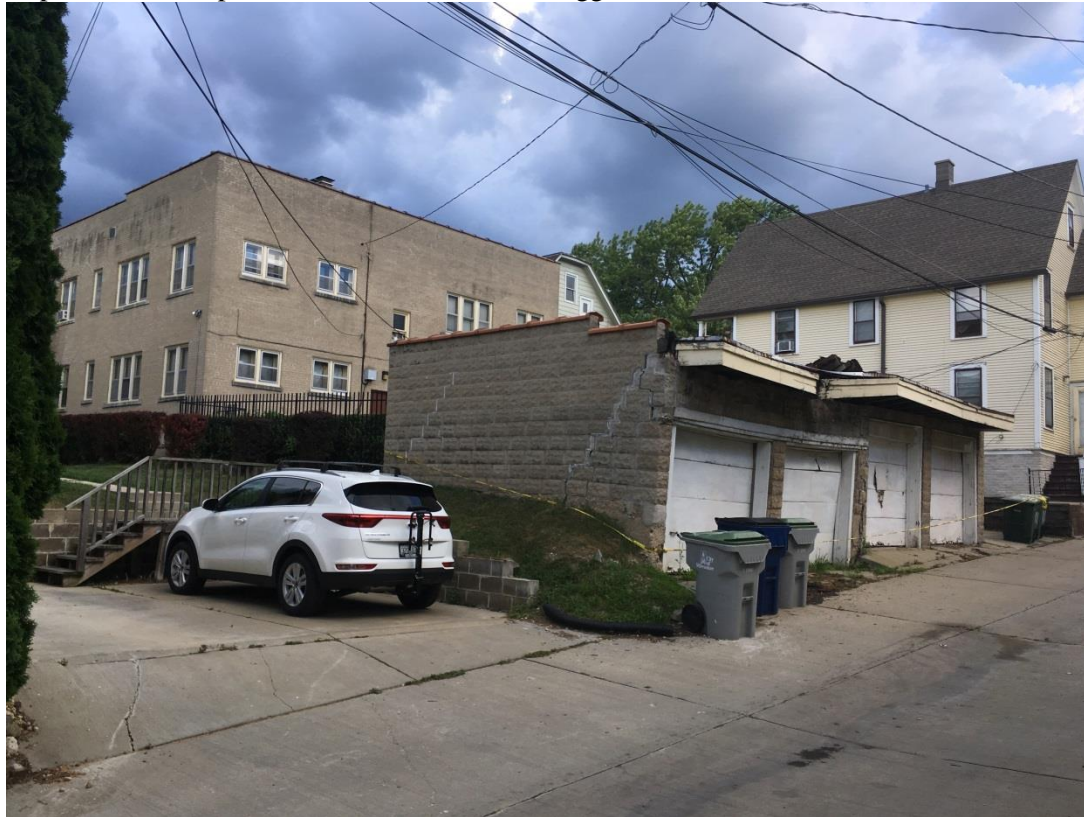
Site conditions showing previous garage.
