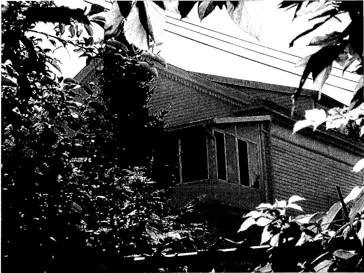
The sunroom as completed
