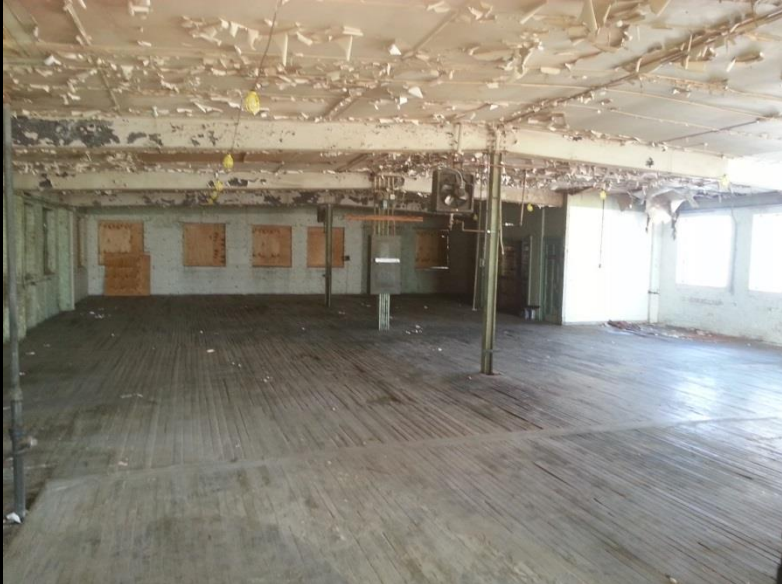
File No. 140044. Interior Photos
