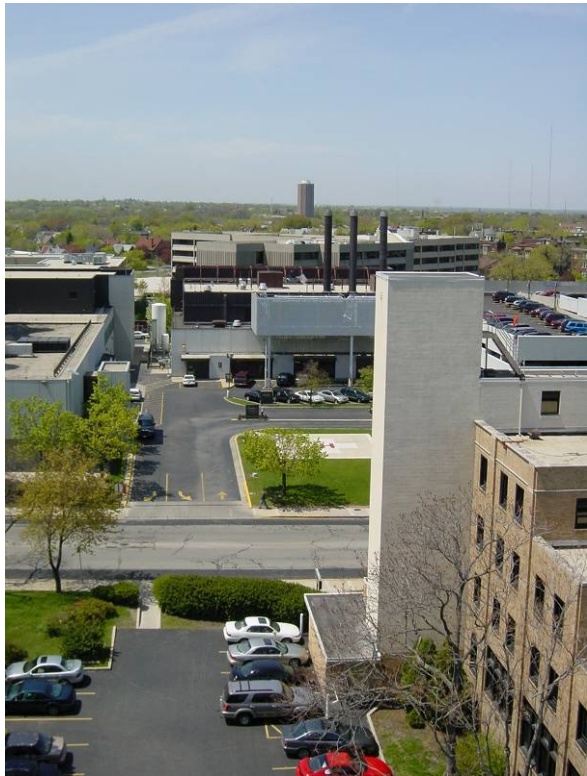
Central Utility Plant
