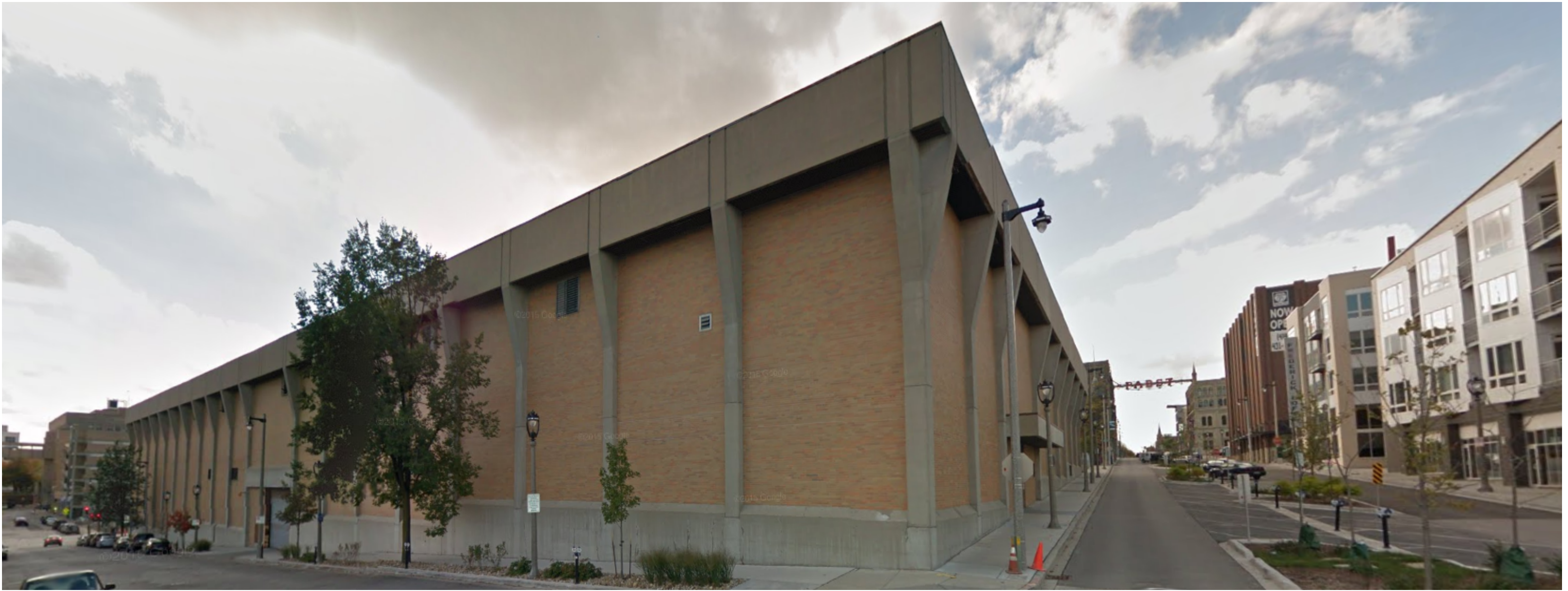
NORTH EAST CORNER
