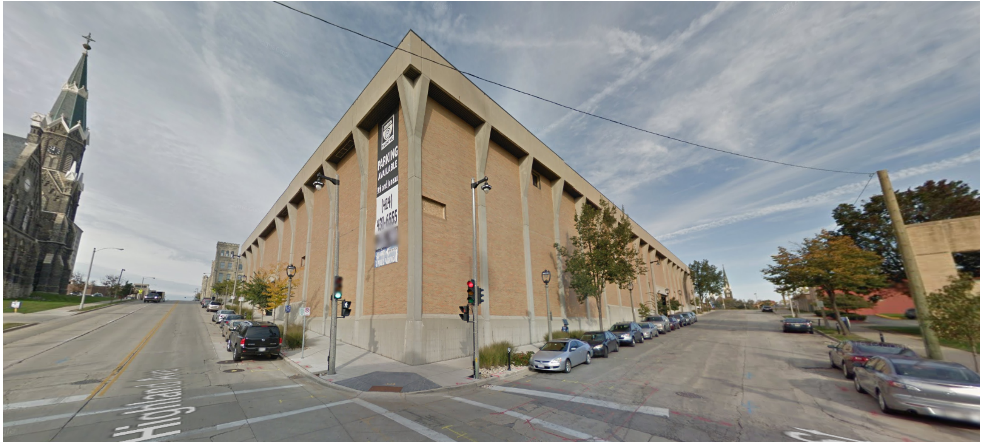
SOUTH EAST CORNER
