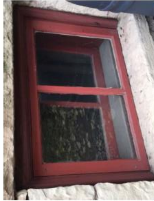
Example of existing 2-pane exterior storm windows on basement
